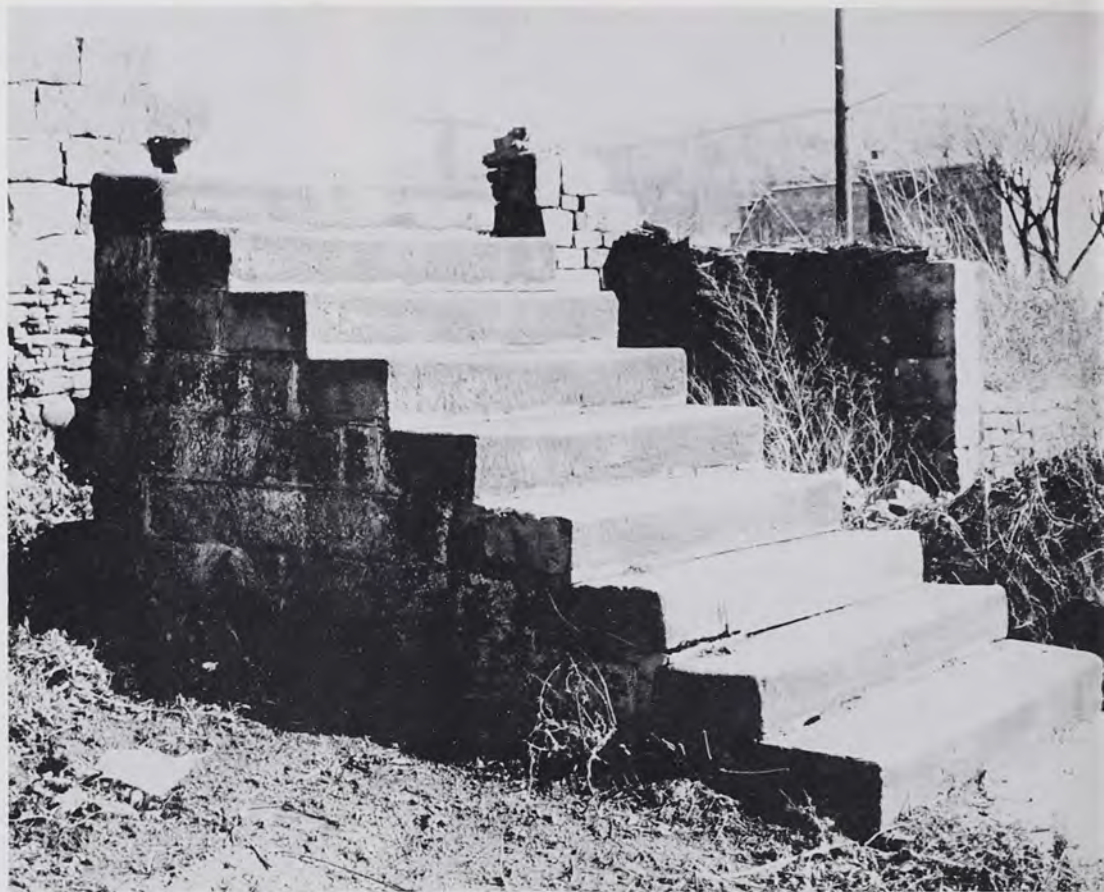
FIG. 6: Front steps. Each step was a six foot long slab of dressed quarried sandstone.
