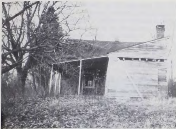
Fig. 9: The rear view of the dwelling shows the extent of the wooden addition as well as the existence of a concrete patio/porch which provided a second entrance to the structure.
