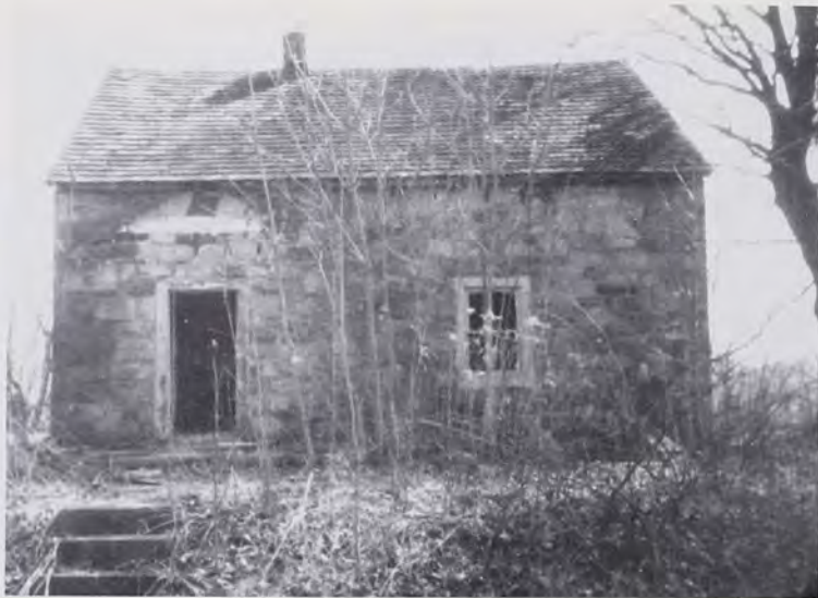
Fig. 7: Front view of the third and most structurally intact stone tenant structure on the grounds of present-day Elizabeth Farms. This Flürkuchenhaus , or half kitchen house, is located on Farm Number Two and is the structure under discussion in this study. Note the asymmetrical front appearance and off-center central chimney. This latter characteristic has given the architectural form its more common name—the Central Chimney house type.
