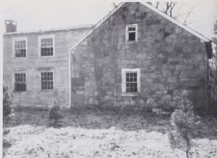
Fig. 8: The left side of the dwelling also shows architectural elements common to people of German-speaking culture including overhanging rafter projection (which can be seen along the front face) and symmetrical window placement on the gable end. Also note the existence of the dependent wooden addition, with its own chimney, to the rear of the main stone dwelling.
