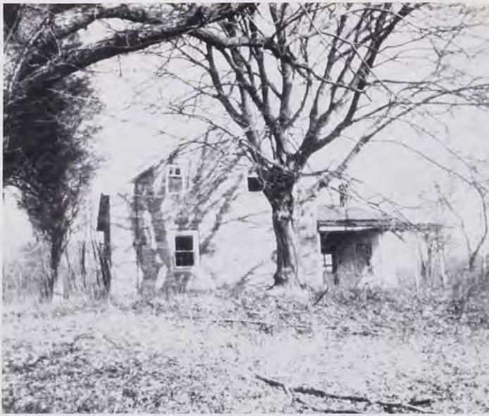
Fig. 11: The right side of the structure, like the left, exhibits architectural elements common to people of German-speaking culture including overhanging rafter projection (here seen along the front and rear faces of the dwelling) and symmetrical window placement on the second level of the gable end. Also note that the wooden addition provides a new doorway and gives access to the former Küche area (now serving as an English Georgian-style hall) from the rear.
