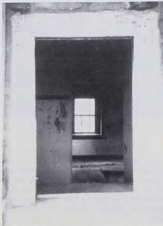
Fig. 10: This close-up of the rear window of the first floor Kammer , located at the rear of the stone portion of the structure, shows that it was placed opposite the front window, located in the Stube , and in line with the only connecting doorway to allow for maximum ventilation.
