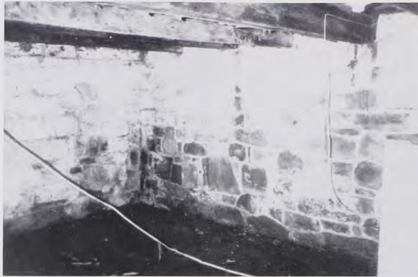
Fig. 15: This view of the cellar shows the massive ceiling beams which could be packed with mud and straw to provide insulation for food storage. Note, too, that the floor is dirt.
