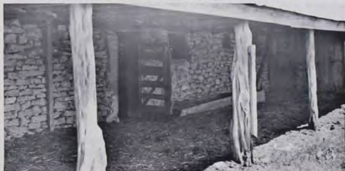
Figure 9: Beneath the forebay of the Hamic barn, viewed from the barnyard. Note the cedar support posts. Photo 1979 by the author.
