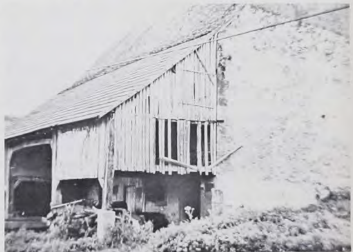
False forebay, Village of Lorenzen, France, near the border with the German Palatinate. 1978.
