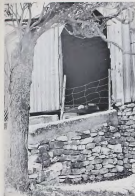
Figure 6: North side of the bank, Hamic barn. Photo 1979 by the author.
