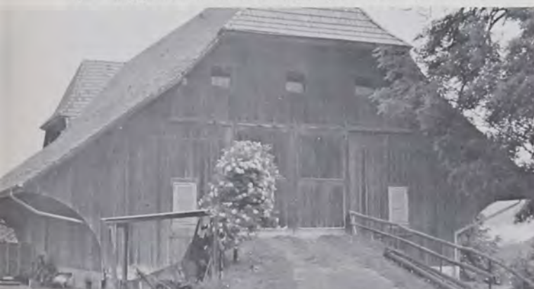
Figure 7: Barn in the Swiss Hamlet of Fahrni, Canton Bern. Note the gable-end bank and the partially-hipped roof. The overhanging eave closely resembles a forebay. This hamlet is reputedly the ancestral home of some eighteenth-century Pennsylvania German emigrants. Photo 1978 by the author.
