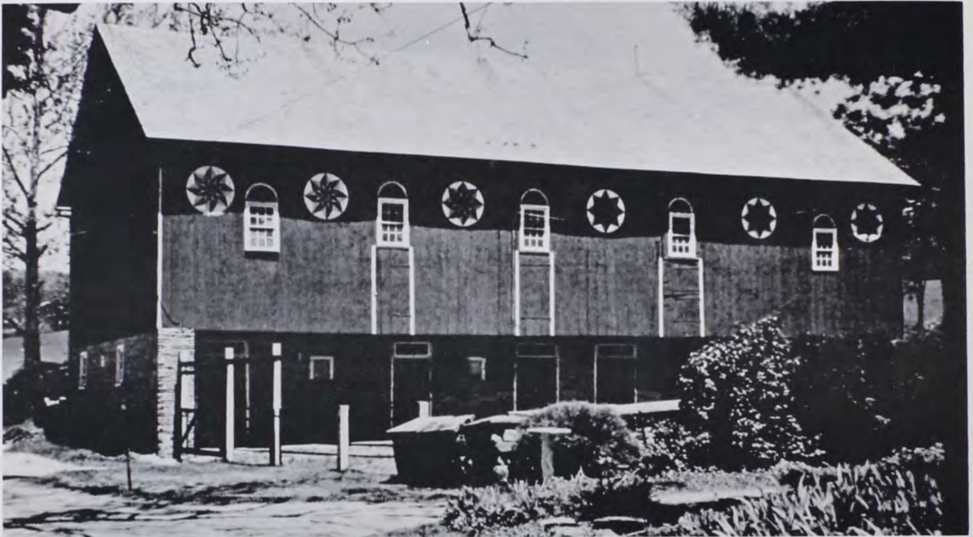
Leiby barn, 1871, Lehigh County, PA. Typical nineteenth century Pennsylvania Barn with forebay supported by extension of basement walls. This barn photo 1975 by author, as all other contemporary barn photographs.
