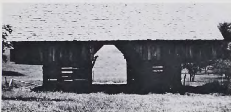
Transverse crib barn or "cantilever," Cades Cove, Great Smoky Mountains National Park, TENN. 1977.
