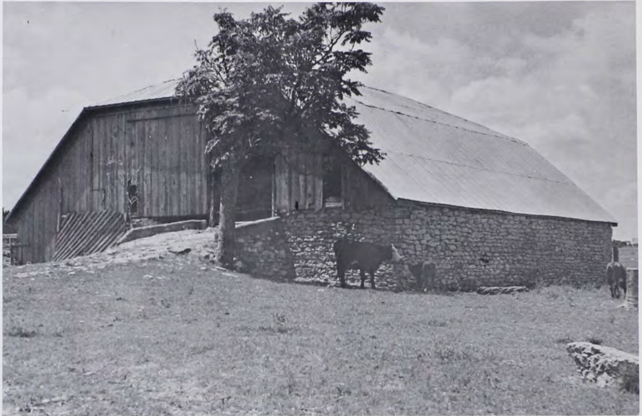
Figure 1: The Hamic barn, northeast elevation. Photo 1979 by the author.
