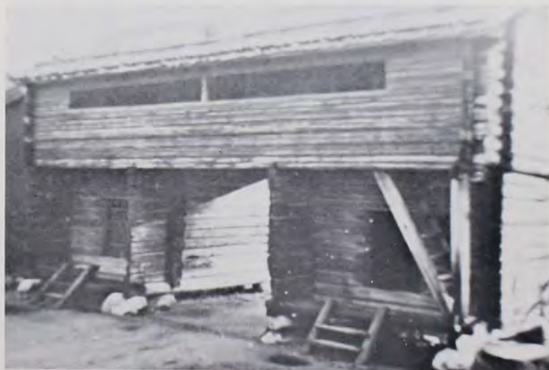
Swedish log pen barn with cantilevered overhang, located in the Outdoor Museum at Sigtuna, Sweden.
