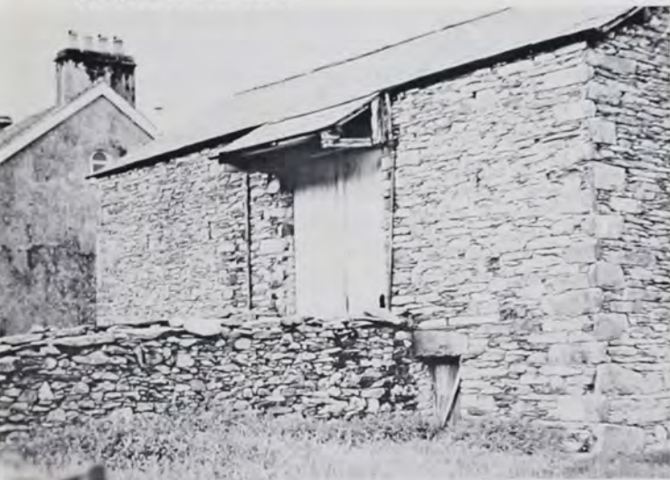
English bank barn, ramp to loft, Southern Lake District, England. 1978.
