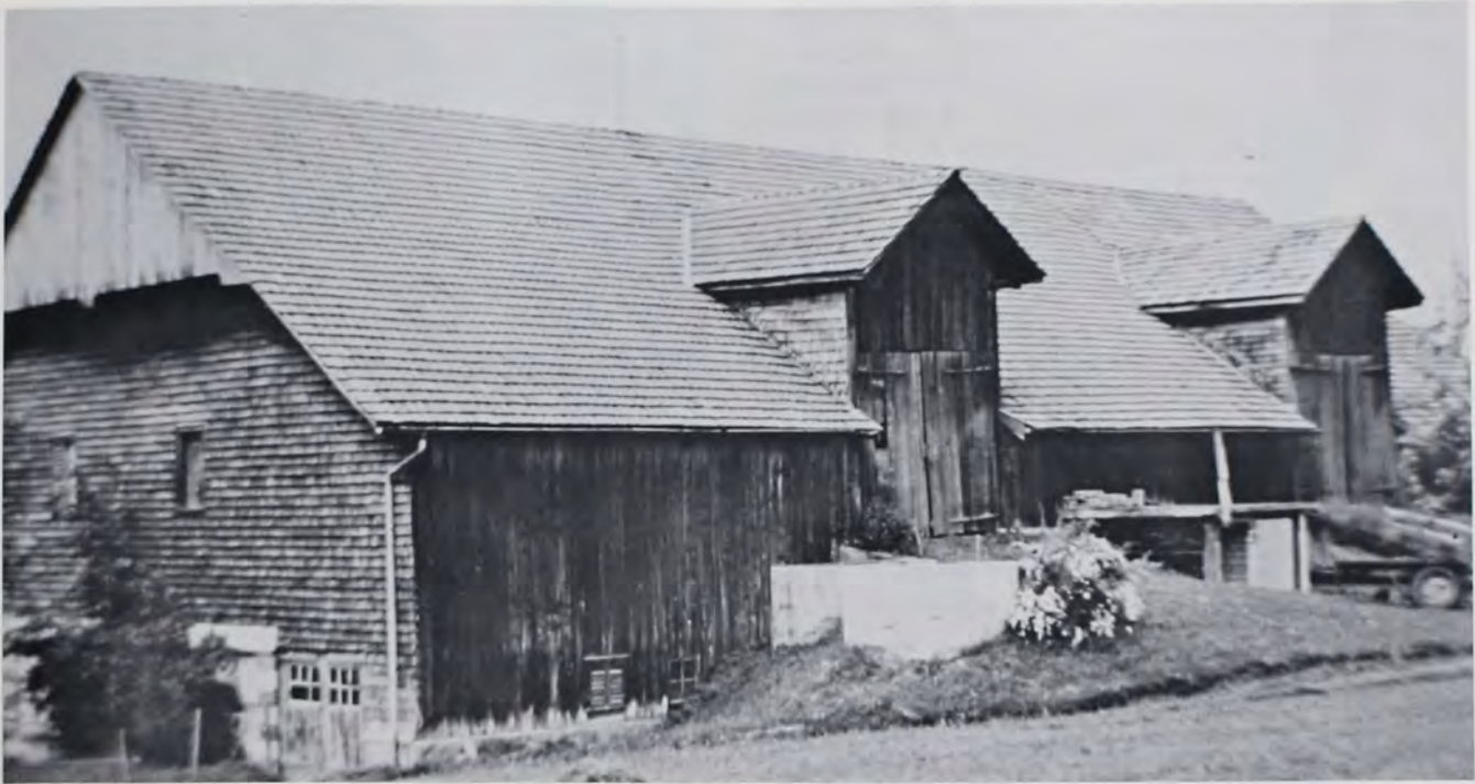
Entlebuch, Canton Lucerne, Switzerland: large two-ramp forebay barn. 1978.
