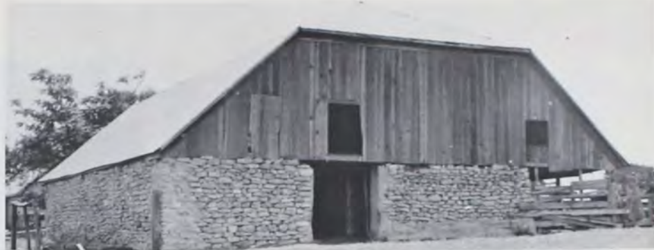
Figure 8: Northwest elevation of the Hamic barn, showing the forebay, to the right, and the partially-hipped gambrel roof. The large opening in the lower level lacks a door. Photo 1979 by the author.
