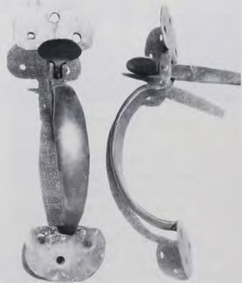
Suffolk latch with bean cusp; this was the most widely used design. (Sorber Collection)
