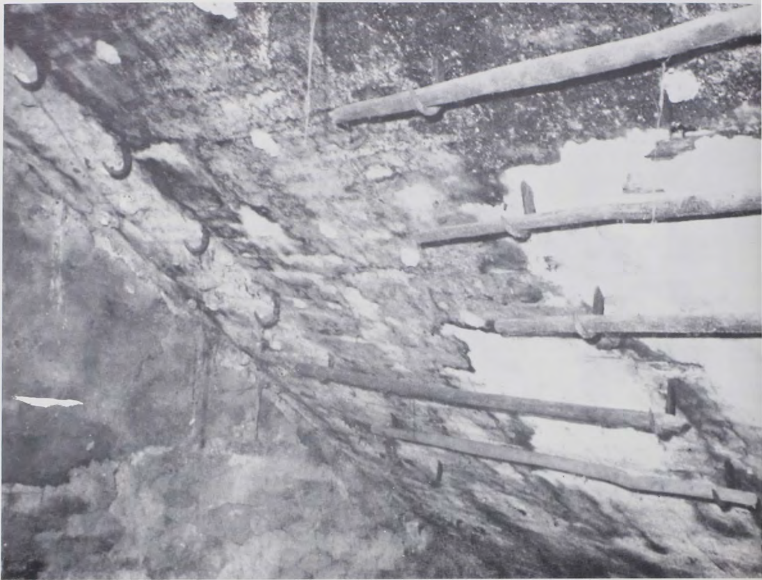
Figure 8. Detail of the hooks and hickory rods in the ceiling of the Rauchkammer.
