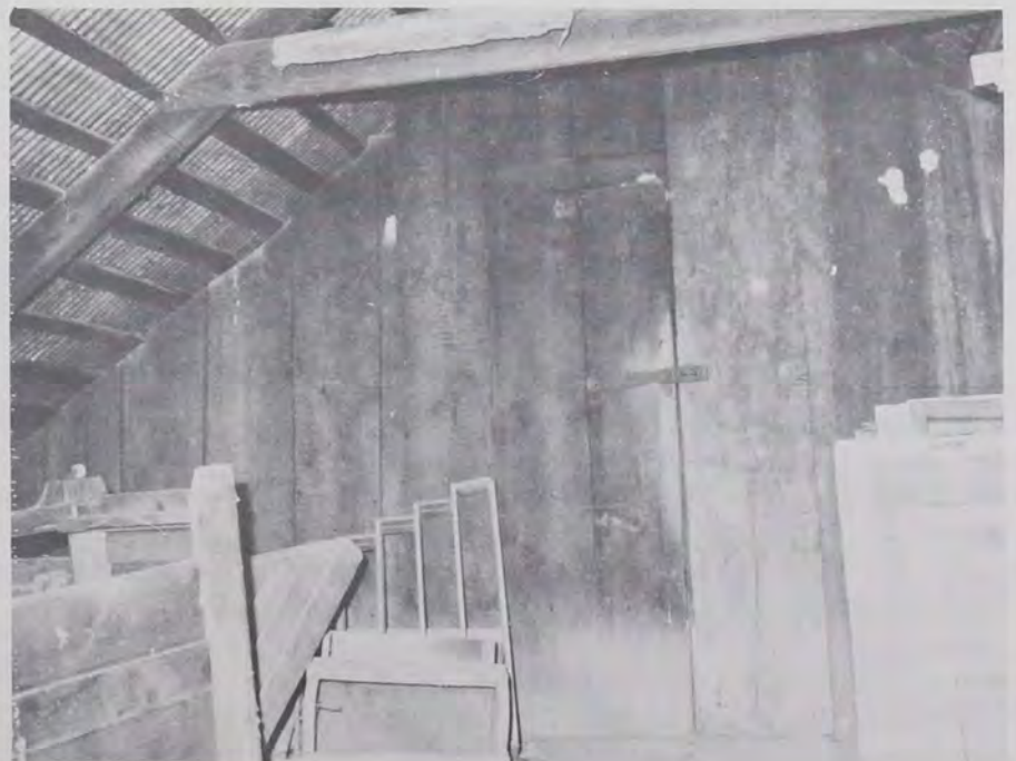
Figure 7. Looking East toward the partition wall of the Rauchkammer.
