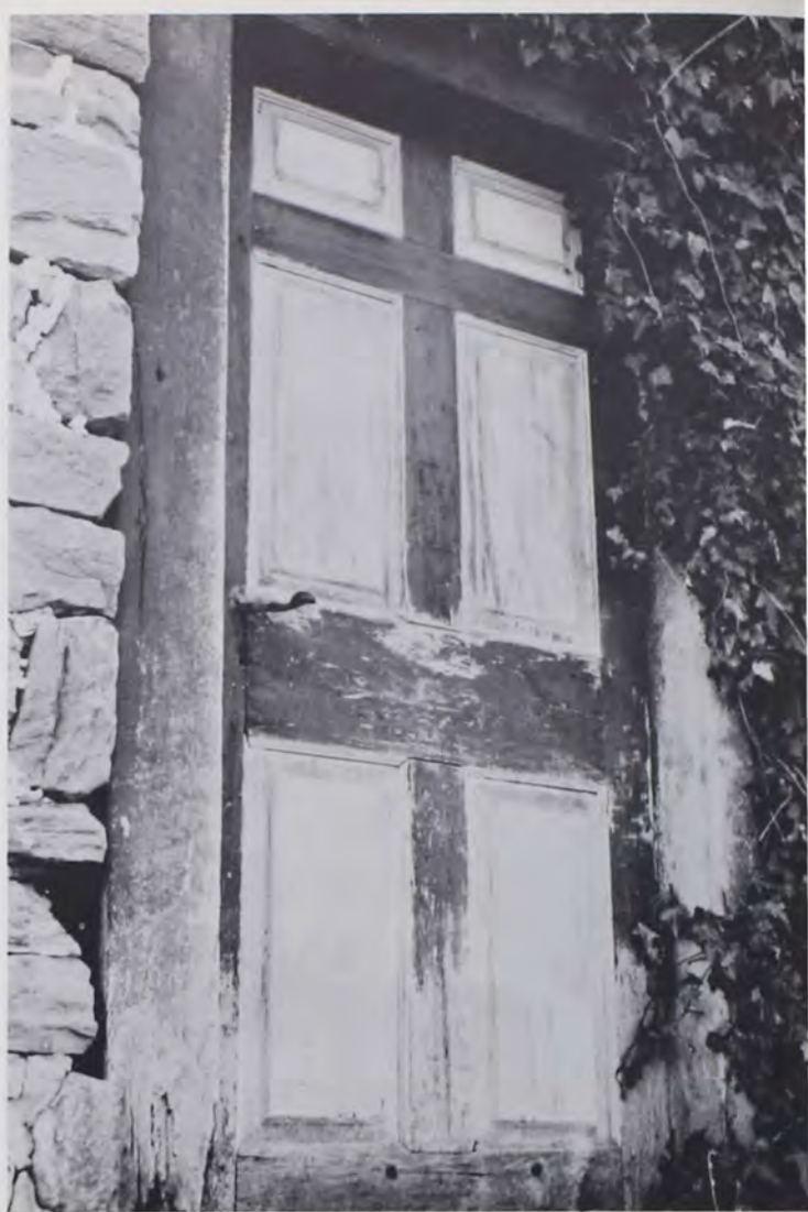
Figure 5. Detail showing the early 18th-century door on the North facade of the Hauser kitchen. Note the antique thumb-latch.
