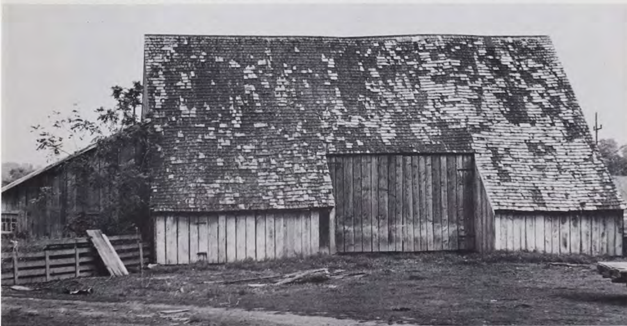
FIG. 12—Double-Crib Barn Subtype II. This barn is located north of Williams- port, Washington County, Maryland. One of the cribs is of V-notched log and serves as stabling, the other is frame and serves as a hay mow. The sheds flanking the large doors are unusual on one-level barns, although frequently found on the large two-level Pennsylvania barns. For the floorplan see Fig. 8C (August, 1965).
