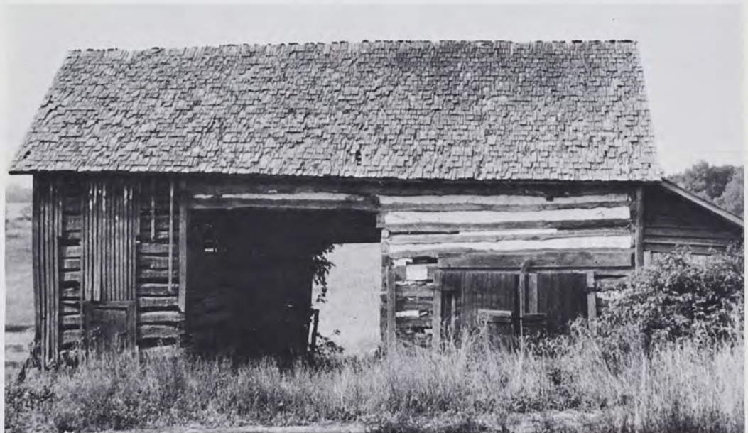
FIG. 12—Double-Crib Barn Subtype II. This barn is located north of Williams- port, Washington County, Maryland. One of the cribs is of V-notched log and serves as stabling, the other is frame and serves as a hay mow. The sheds flanking the large doors are unusual on one-level barns, although frequently found on the large two-level Pennsylvania barns. For the floorplan see Fig. 8C (August, 1965).
