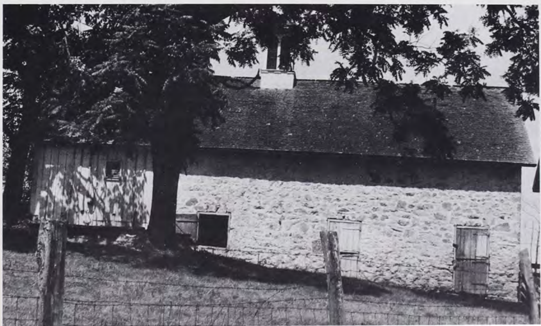
FIG. 3—Stone Type A, C Barn. This is located near Burtonsville, Montgomery County, Maryland. The door to the hay loft is located on the opposite side. The frame end addition was built in mid-19th Century, probably about one hundred years after the stone barn. The stone barn measures 28' x 40'. For the floorplan see Fig. 1E.
