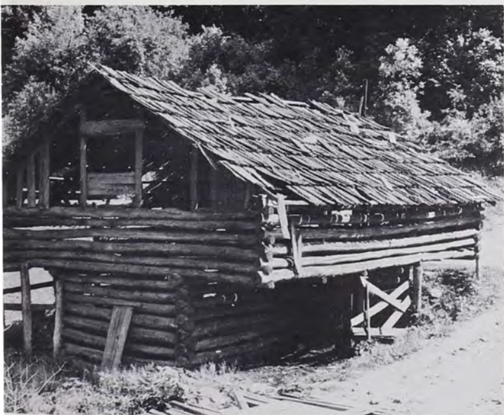
FIG. 19—Double-Crib Barn with Cantilevered, Overhanging Loft. This V-notched barn is located east of Selbiana, Pike County, Kentucky. The floorplan is like Fig. 17B, except that the doors of each crib open into the runway (June, 1964).
