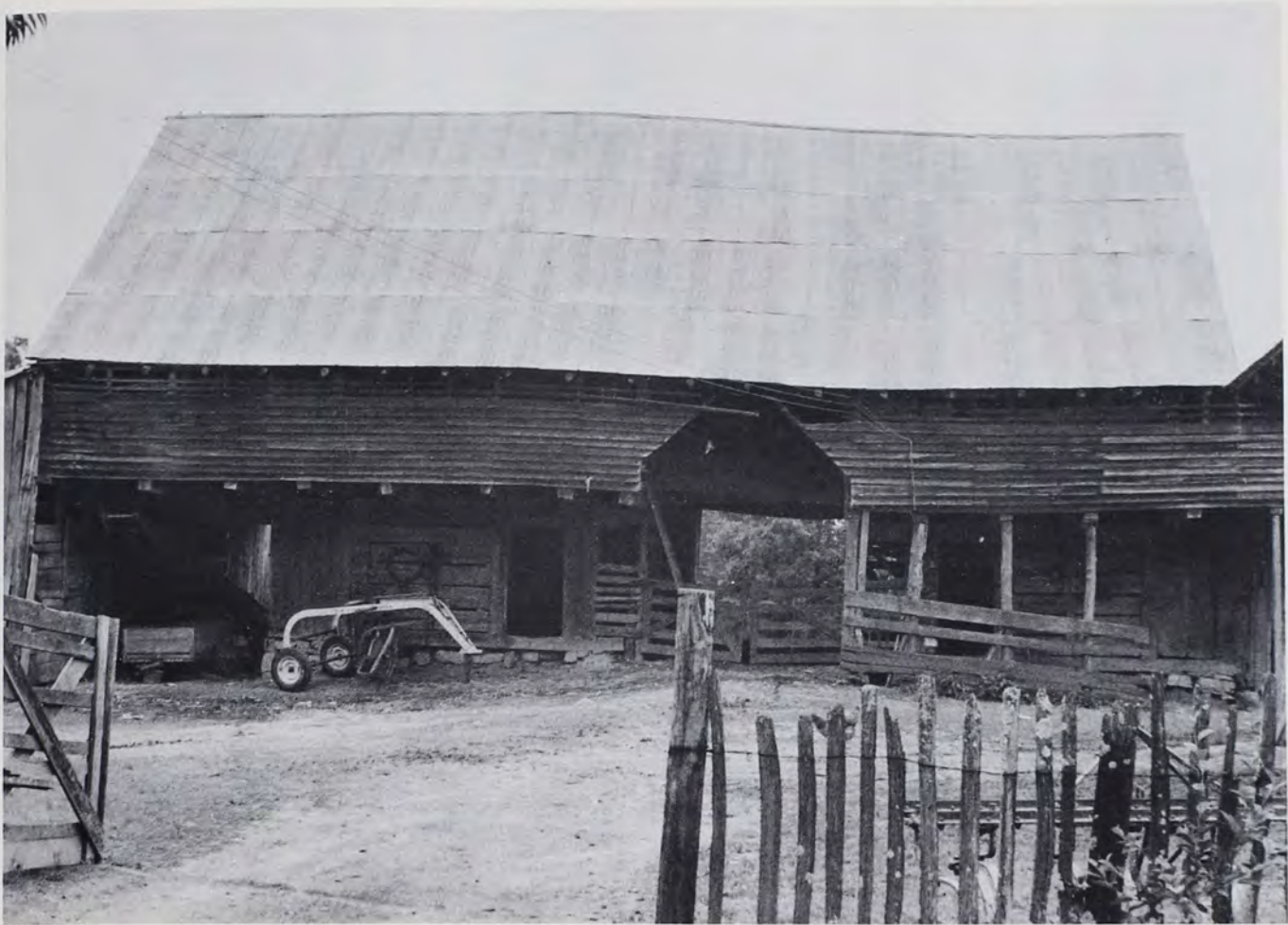
FIG. 18—Double-Crib Barn with Cantilevered, Overhanging Loft. This barn is located north of Marysville, Blount County, Tennessee. The frame loft of this barn overhangs on all four sides. The log cribs, which have the logs tenoned into corner posts in the front and V-notched in the rear, measure 23' x 16'. For the floor-plan see Fig. 17C (May, 1964).
