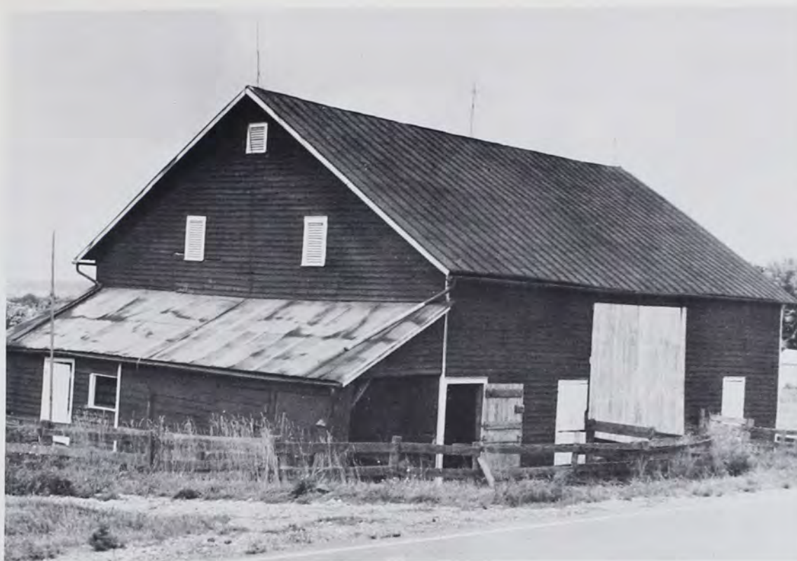
FIG. 5—Type D. The English or Connecticut Barn. Located between Grottoes and Dooms, Augusta County, Virginia. This barn has the same louvers, red painted clapboards, and white trim as the two-level (type F-J) Pennsylvania barns in the same area (July, 1964).
