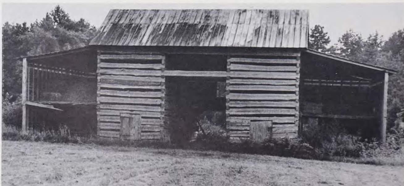
FIG. 9—Double-Crib Barn Subtype II. This half-dovetail log barn is located south of Faith, Rowan County, North Carolina. The cribs are employed for stabling, have a large hay mow, and measure 12' x 20'. The sheds on the side are for the storage of farm machinery, that in the rear is divided into stalls with one section set aside for chickens. For the floorplan see Fig. 8A (August, 1965).
