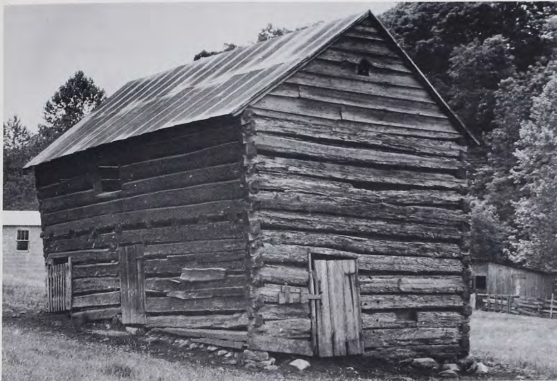
FIG. 2—Type A, C Barn of Half-Dove-tailed Log. This is located near Rock Oak, Hampshire County, West Virginia. For the floorplan see Fig. 1D (June, 1964).
