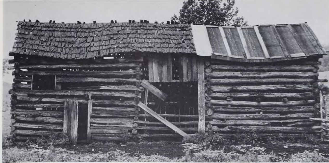
FIG. 10—Double-Crib Barn Subtype II. This barn is located southwest of Cran- don, Bland County, Virginia. The roughly V-notched cribs are used for stabling and are 11 feet square. See Fig. 8F for the floorplan (July, 1964).
