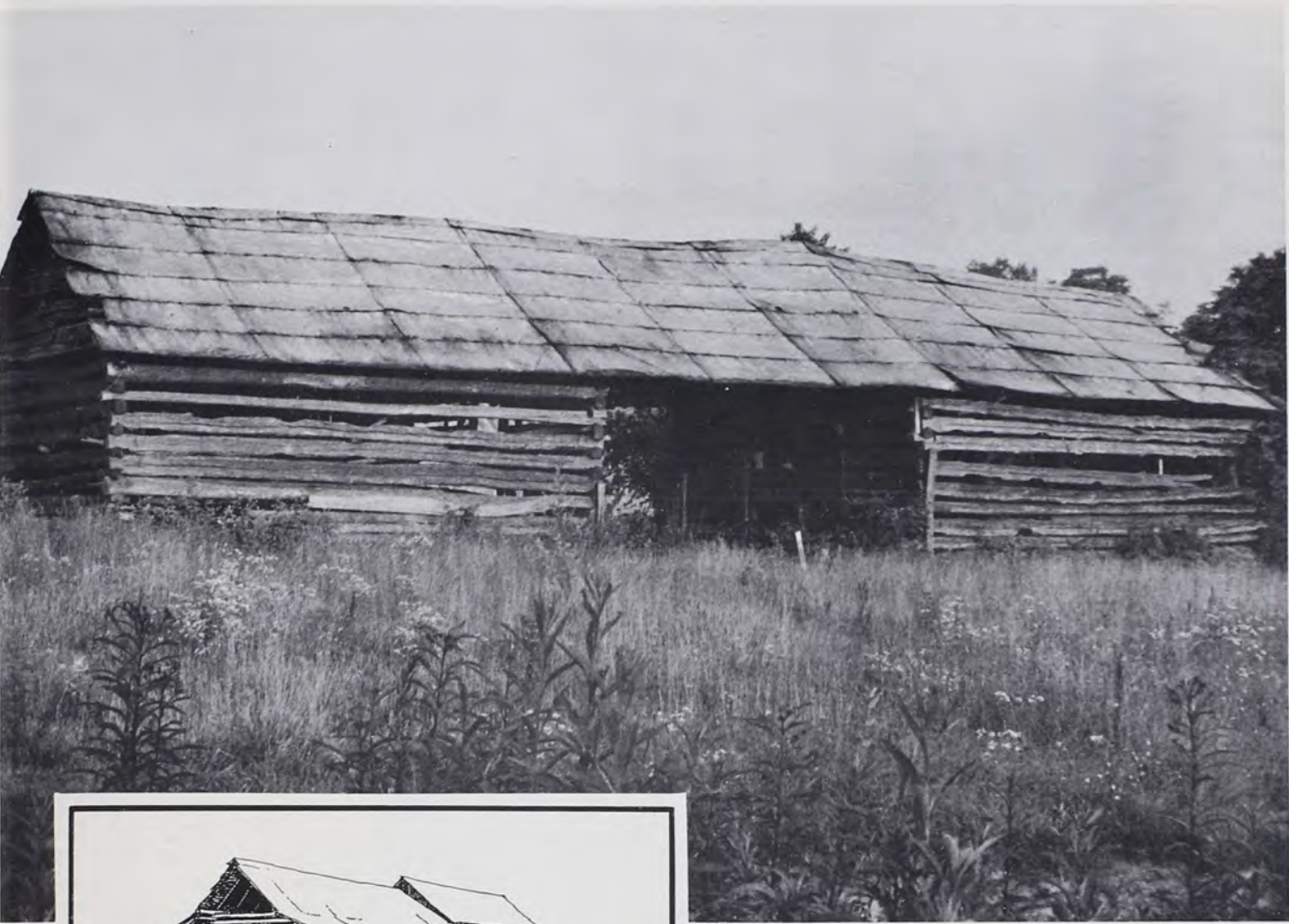
FIG. 7—Double-Crib Barn Subtype I. This V-notched log barn is located northeast of Bristol, Washington County, Virginia. For the floorplan see Fig. 6D (July, 1964).
