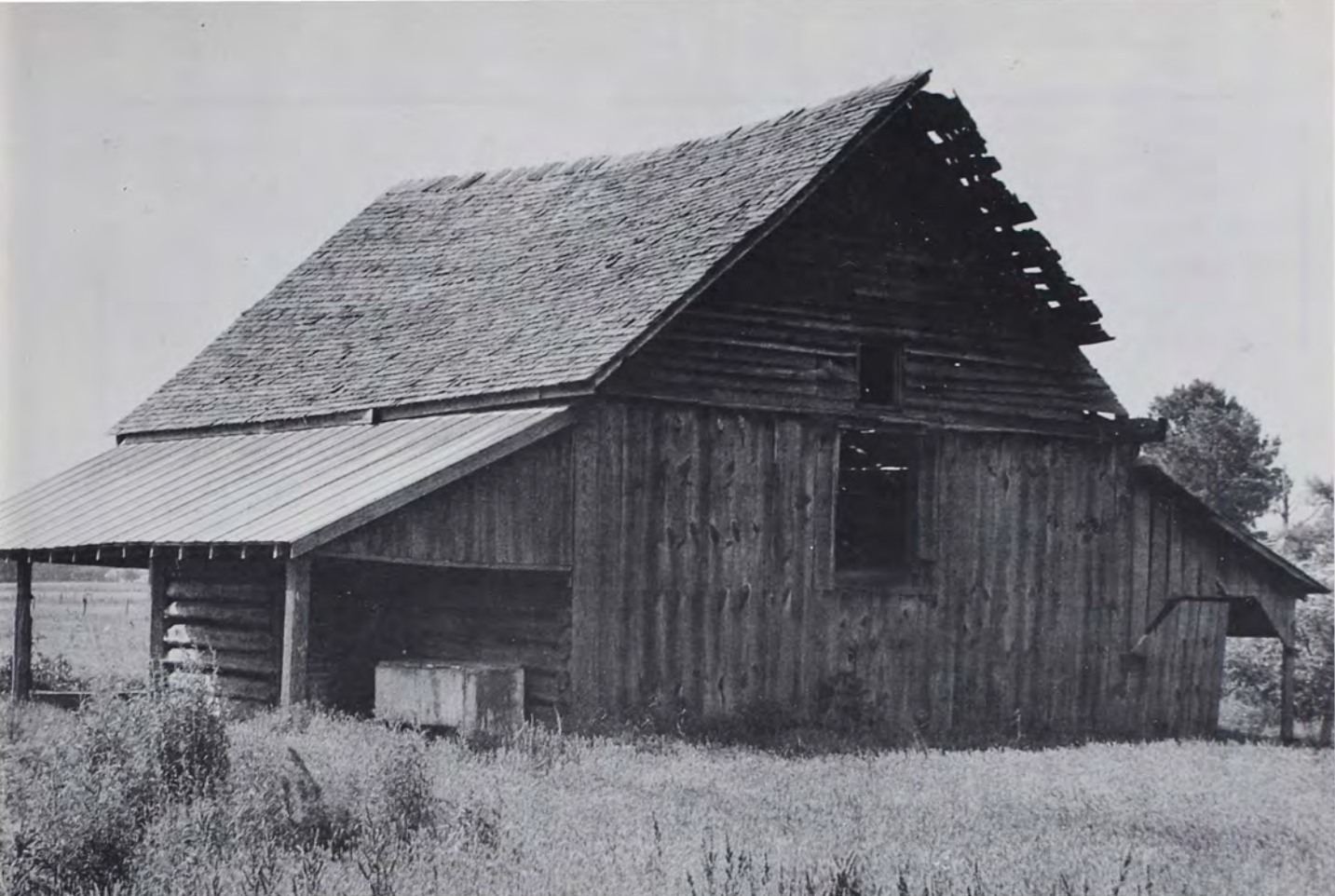
FIG. 14—Double-Crib Barn Subtype III. This barn is located southwest of Walnut Grove, Blount County, Alabama. Its V-notched cribs measure 10' x 25'. See Fig. 13C for the floorplan of this barn (May, 1964).
