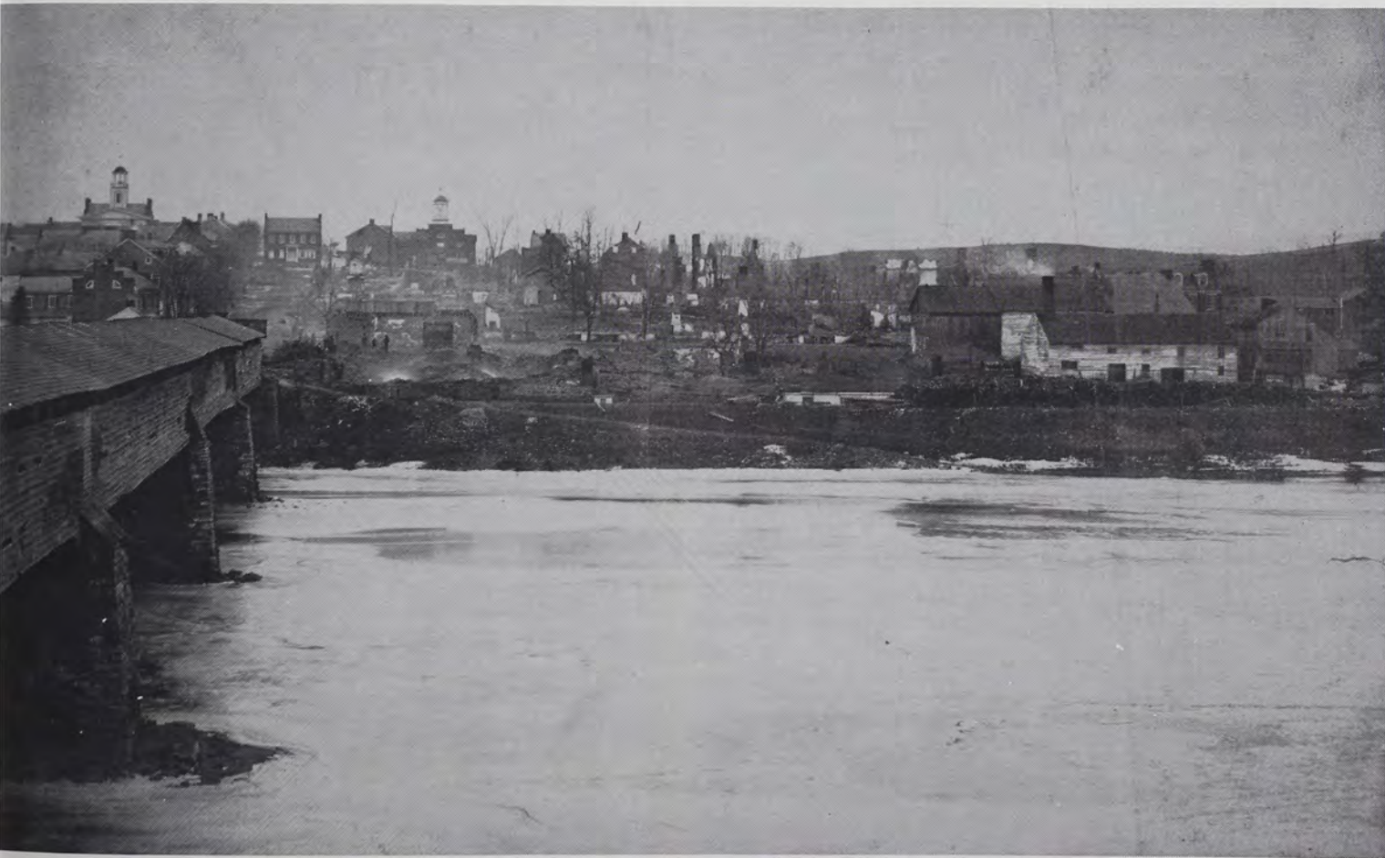
Figure 8. Mifflintown, Juniata County, Pennsylvania, after the fire of December 31, 1870. Note immense covered bridge across the Juniata River, the courthouse (upper left), Lutheran Church to the right of the bridge line, the huge factory complex, possibly a tannery from the piles of wood or bark, and the obvious devastation wrought by the fire, which left only chimneys standing on many house sites. The fire can be seen smoldering along the river to the right of the bridge.
