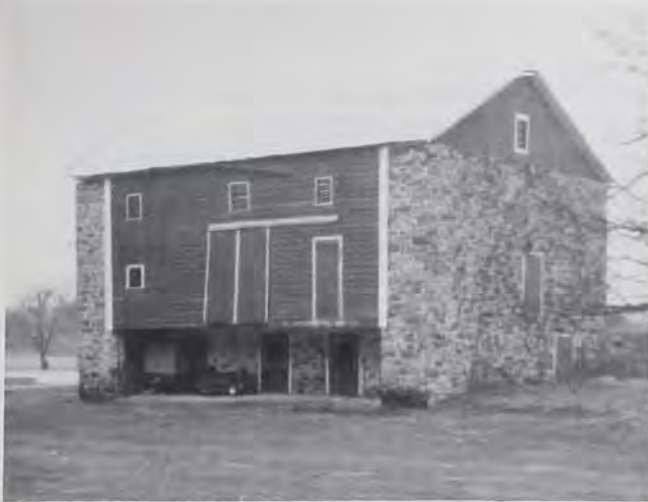
Class II closed forebay standard Pennsylvania barn (ca. 1820) in Harmony Township, Warren County, N.J. has a symmetrical gable-end silhouette, and a fully supported forebay with a pier corner or alcove, a very distinctive feature.
