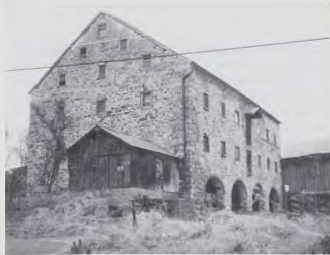
Class III vertical extension ("double-decker") Pennsylvania barn (1816) in Warren County, N.J. has a symmetrical gable-end silhouette, and a fully supported forebay. The top level has a wide central threshing floor; the middle level a granary surrounded by hay mows, with the bottom level used for stabling livestock.
