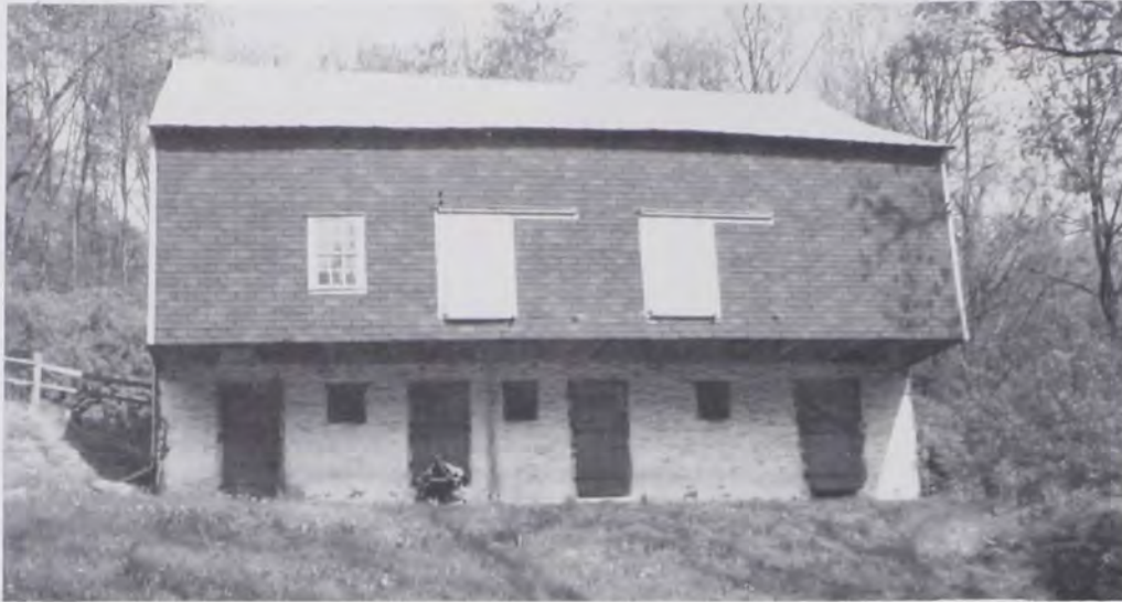
Class I log Sweitzer Pennsylvania barn (ca. 1790-1810) in Greenwich Township, Berks County, Pa., with asymmetrical gable-end silhouette, unsupported forebay, double-log-crib mows separated by a central threshing floor on upper level, and stables below.
