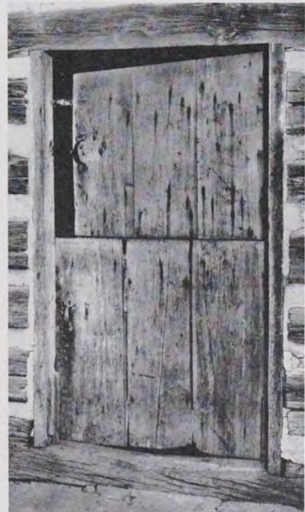
No. 2—The Log House Schneider The "Dutch" door of three beaded boards, bat- tened, reveals excellent iron hardware no doubt made quickly by an ex- pert blacksmith.
