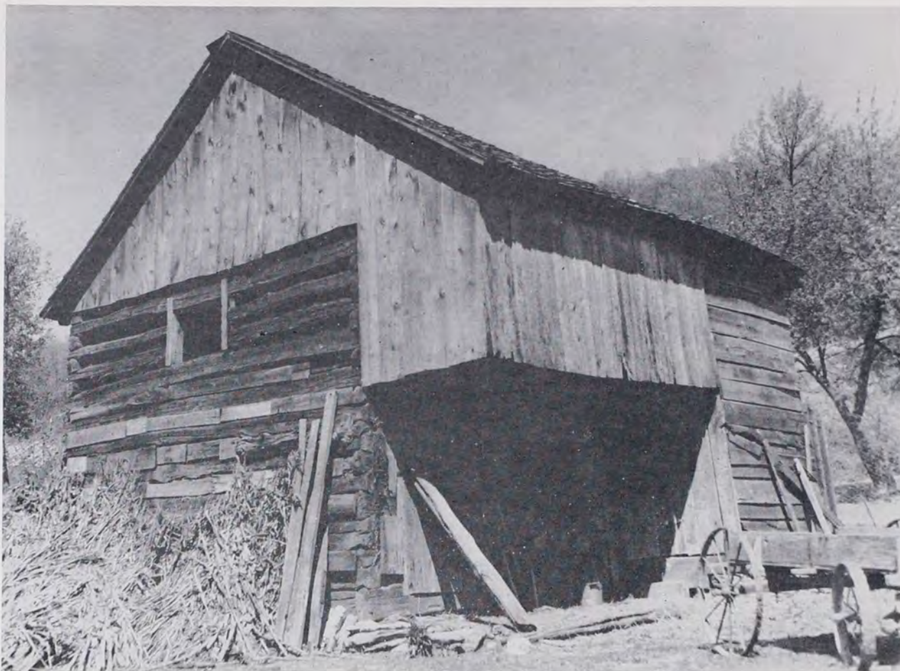
The log barn with a forebay might appear to have been a makeshift but it has served for a long time. There was only one stable and the harness was hung on long wooden pegs on the outside. The small opening at the gable end was for hay storage. The end with the horizontal boarding is a later addition. Located along Route 30 near Chambersburg, Pennsylvania.
