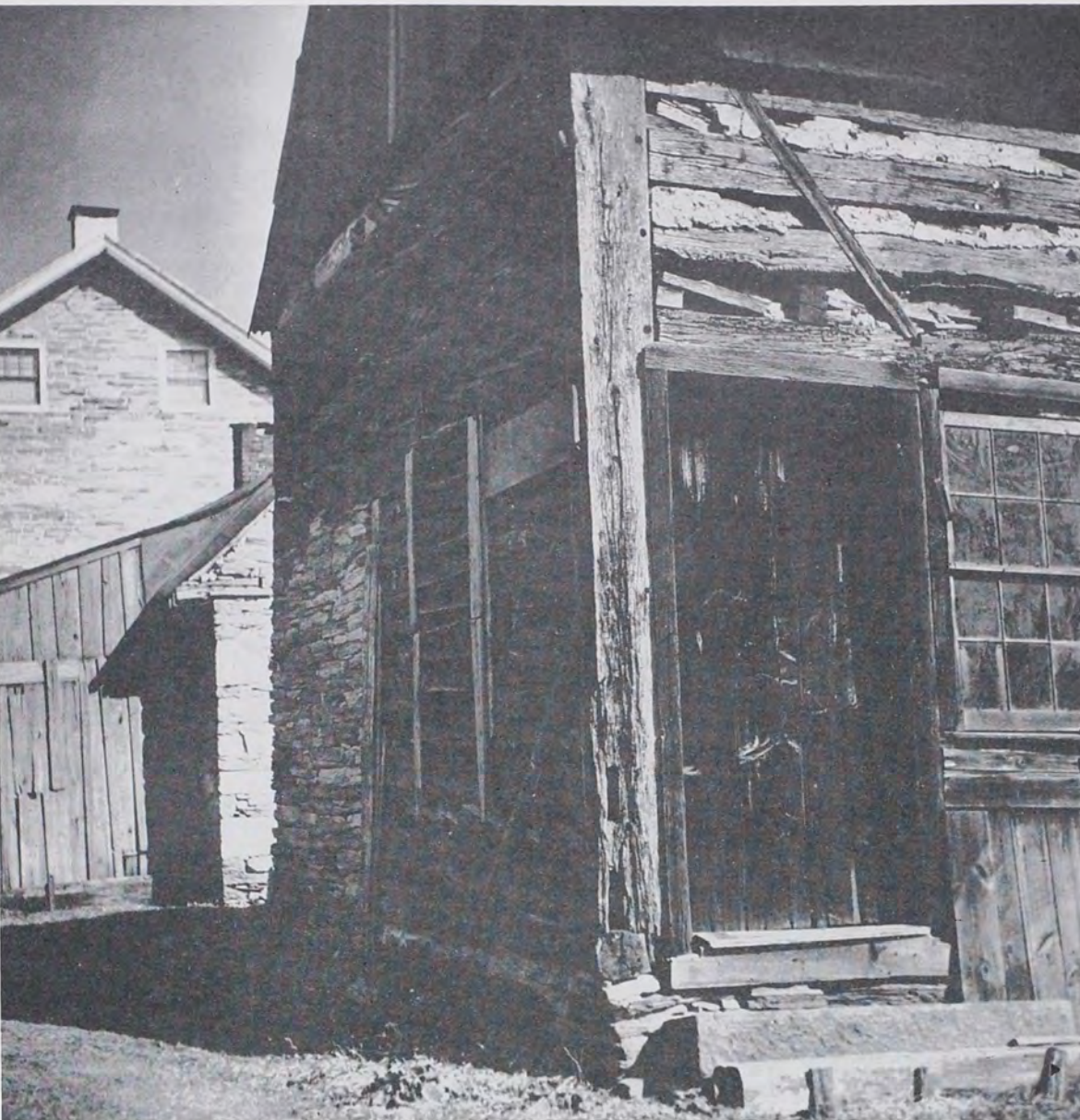
The log house with the vertical corner timber stood at Schaefferstown, Pennsylvania. The horizontal logs were tenoned into the corner log and pinned. This type of corner construction is quite rare for it was obviously very difficult to make.
