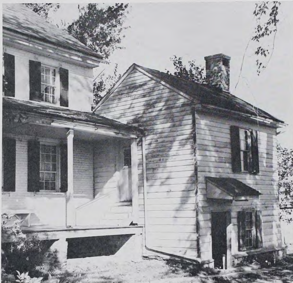
The summer kitchen has a split-level relationship with the balance of the house which was a very functional and attractive arrangement. The clapboard siding is painted white and the shutters dark green. The massive trees in the yard provide a pleasing pattern of shade in the late afternoon.
