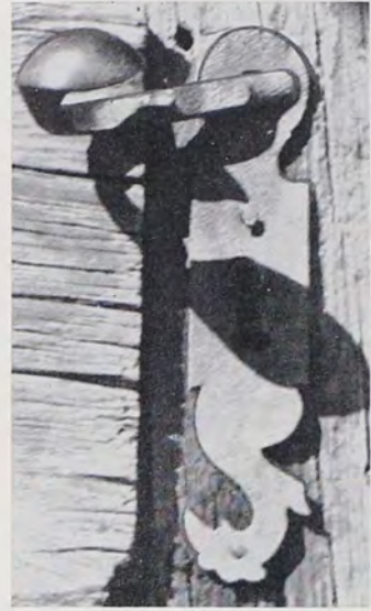
The door has its original press latch with a decorative escutcheon. It appears to be a cock's head turned upside-down.
