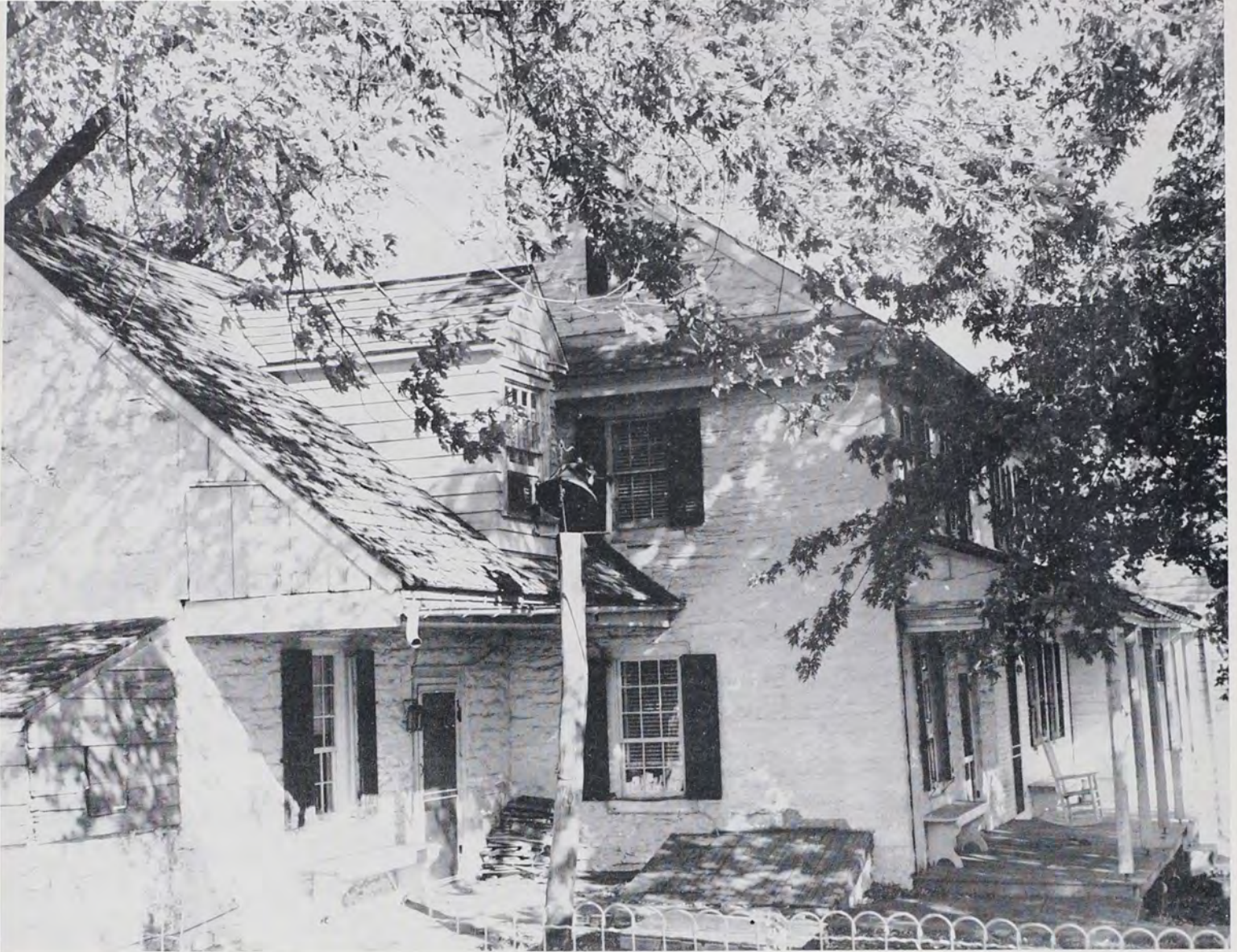
The rear view of the Homestead farmhouse is the most attractive and interesting. The small appendage nearest the camera is the bake oven with its old hand-planed boards and shingle roof. The next part is the farmhouse kitchen with an extending roof to protect the doorway (and some fireplace wood) from the rain. Next is the oldest portion of the house which was built of stone and beyond is the brick addition which was the last major change to the house proper. At the end of the porch, but not otherwise connected with the house, the summer house is located.
