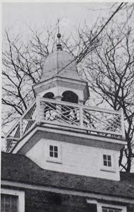
Belfry of the Bell House showing the detail of the Chinese Chippendale railing. This appendage is a masterpiece in plan and execution.
