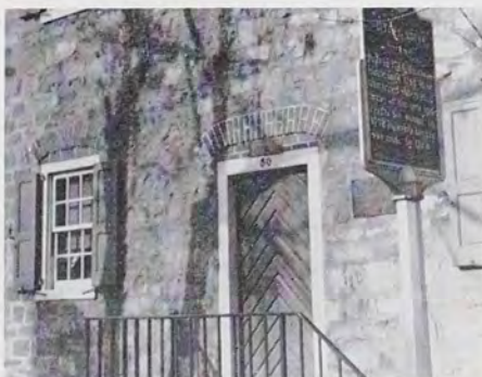
Doorway of the Sister's House. The diagonal mould-joint in the door is found in other spots in Bethlehem.
