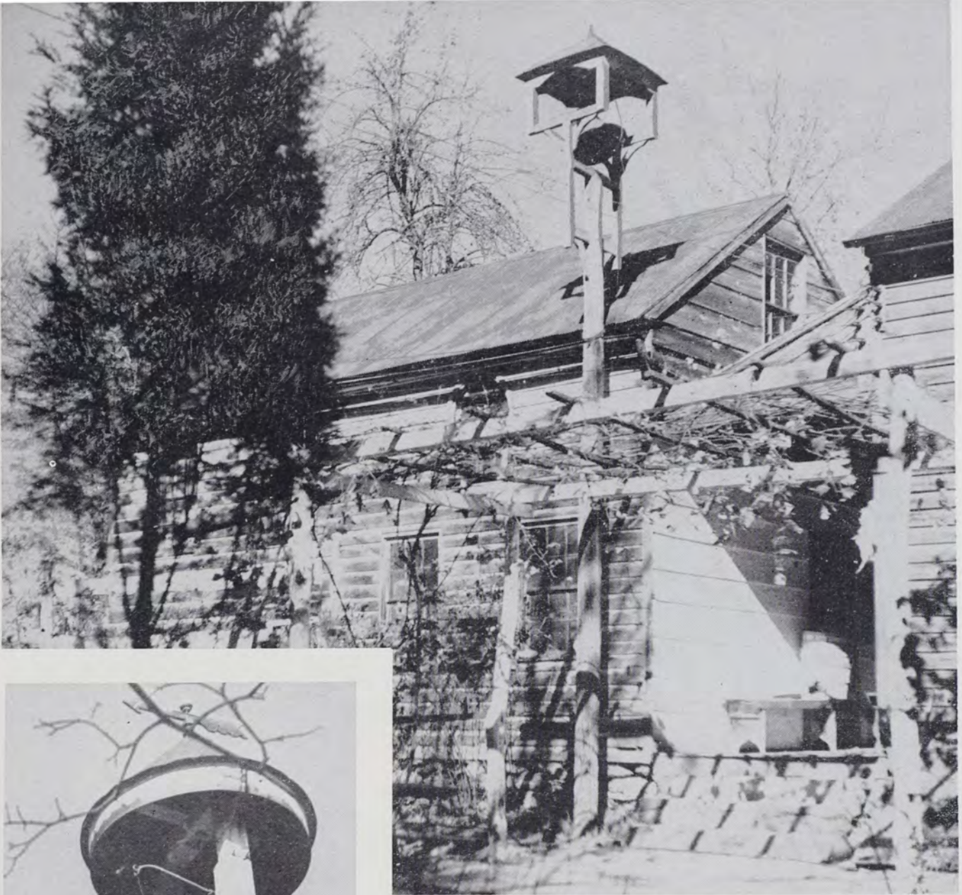
The bell on the pole with its handsome architectural canopy is located in Little Pittsburgh, Lancaster County, Pennsylvania. It was obviously made by an ingenious craftsman for it is both attractive and functional. Very few bell poles have survived for the poles would rot in the ground and due to the scarcity of fine long trees the bell was placed on the house or discarded
