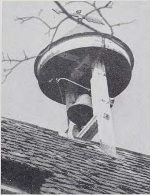
This interesting tower was formerly located on the roof of the Sisters' House at the Ephrata Cloister. The conical roof of sheetmetal and the crude framework of wood indicates that it was not a part of the original structure. The round shape of the roof is extremely rare for bell towers in the Dutch country
