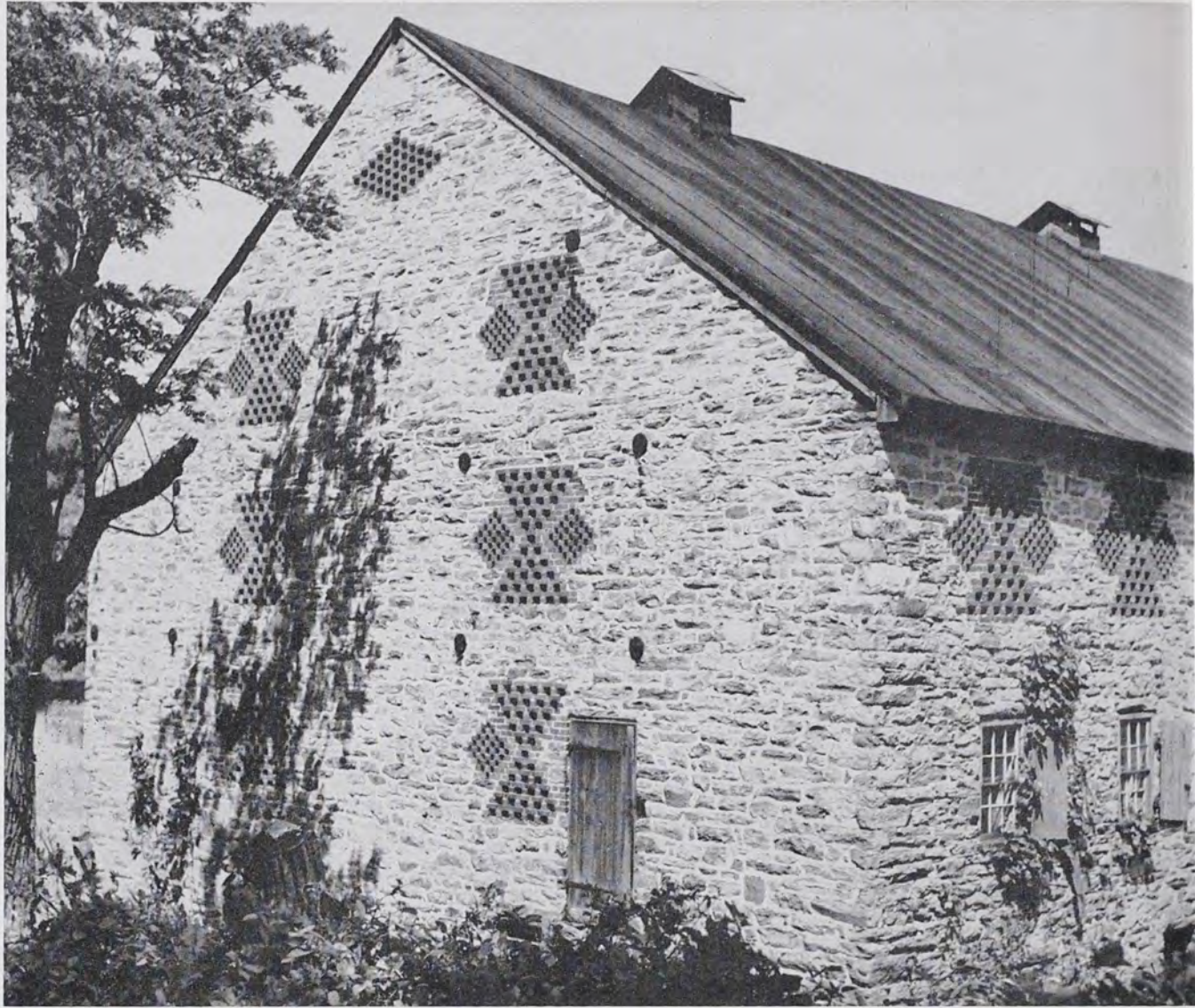
This magnificent example of a stone-end barn with inserted-brickwork designs is on the Gorsuch Farm. This is the finest example of a stone barn having such inserted designs, known to the writer. This barn was owned by the Gorsuch family which precipitated the famous Christiana Riot in Lancaster County in 1851 when members of that family sought to recapture runaway slaves. The barn is located 30 miles south of York, Pa., on Route 111.
