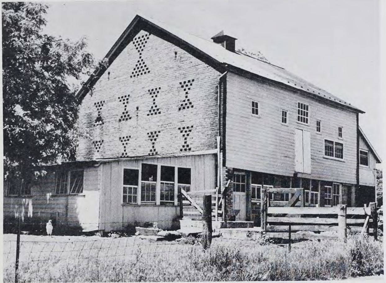
SHEAF-OF-WHEAT DESIGN —This is the only barn known to the writer in which both ends of the barn are decorated with sheaf-of-wheat designs only. The barn is located not far from the old Warrington Friends Meeting House near Wellsville, York County, Pa., on Route 24. This is a relatively small barn.
