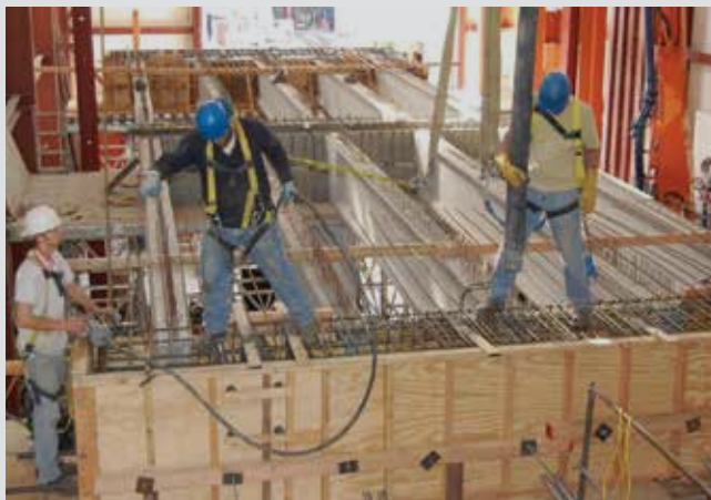
Casting an abutment
