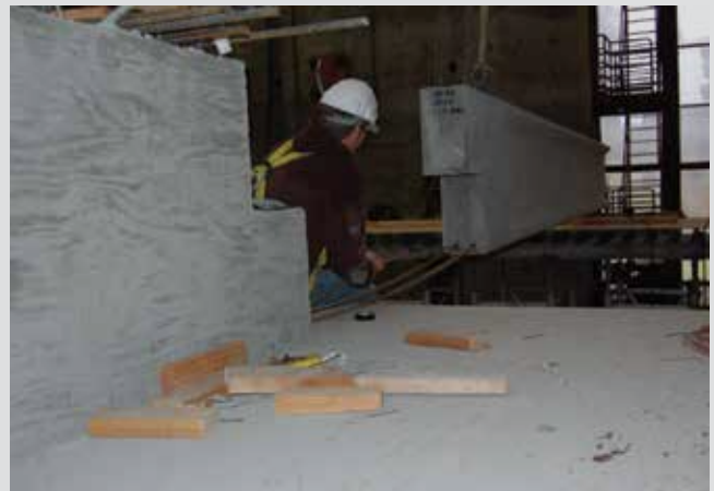
Installing strand for improved girders
