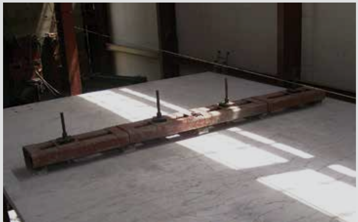
Flexural cracking across the entire deck width
