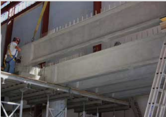
Installing as-built girders
