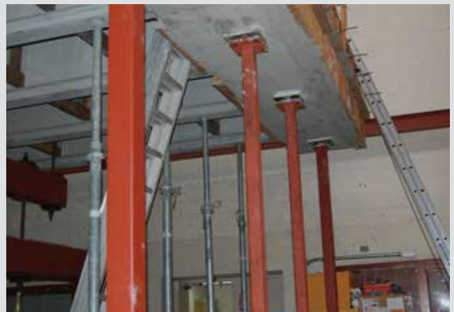
Temporary abutment support
