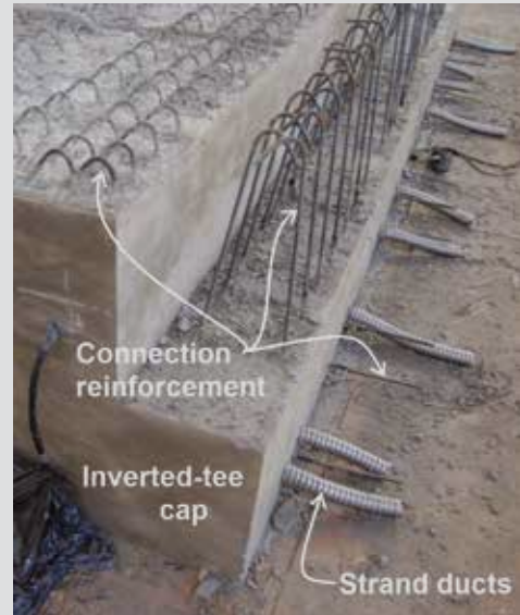
Cap beam prior to girder placement
