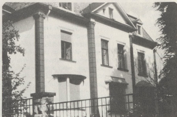
The Goethe Institute in Iserlohn, West Germany.
