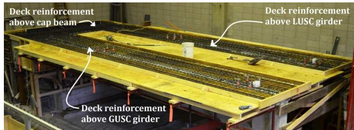
c. Deck formwork and reinforcement
