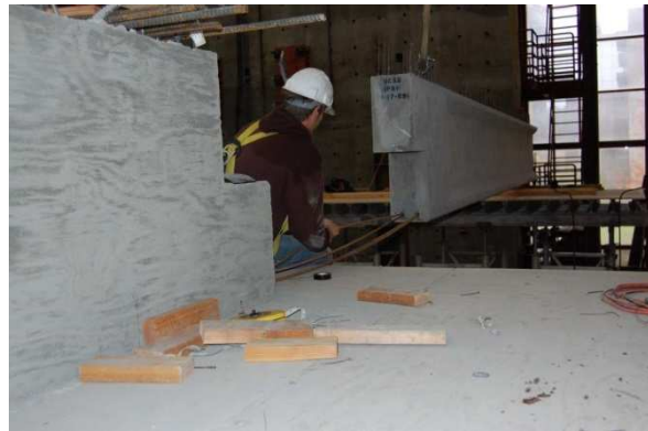
(b) Installing strand for improved girders
