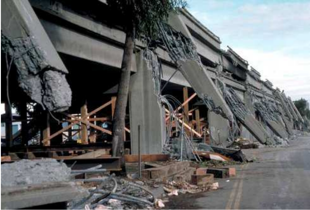
Figure 1.4. Cypress Street viaduct collapse, 1989 (USGS Online Publications Directory, 1999)
