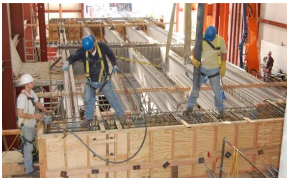
(c) Casting an abutment
