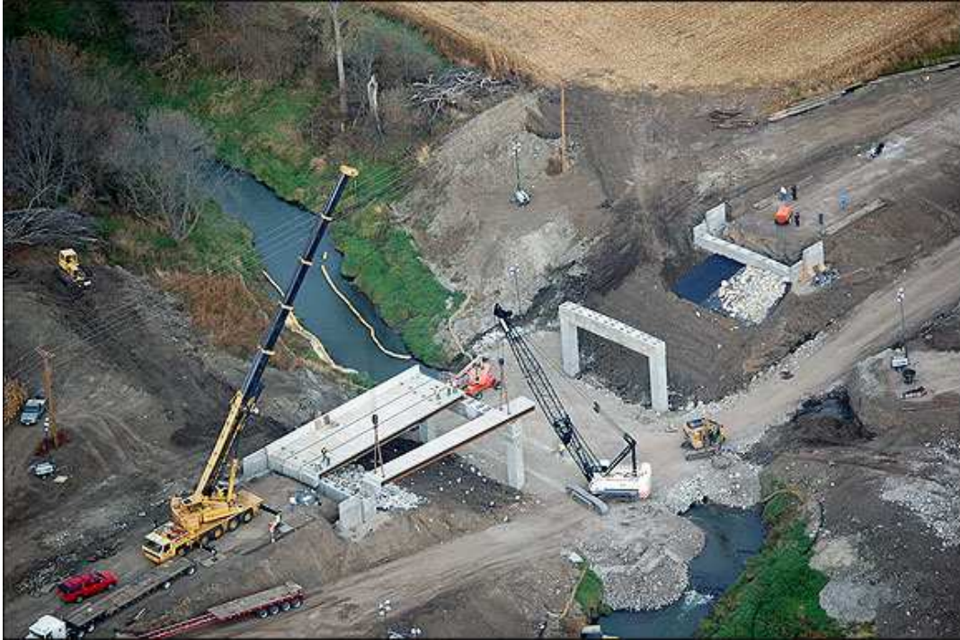
Figure 1.5. Keg Creek Bridge constructed using ABC methods (AASHTO, 2011)
