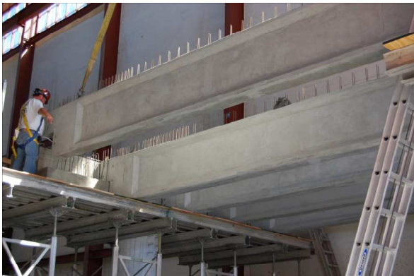
(a) Installing as-built girders
