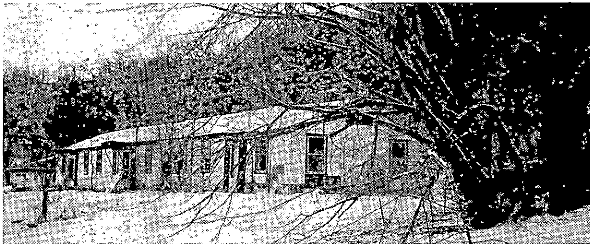
The existing Mankato Barracks, out by the Red Jacket Bridge
