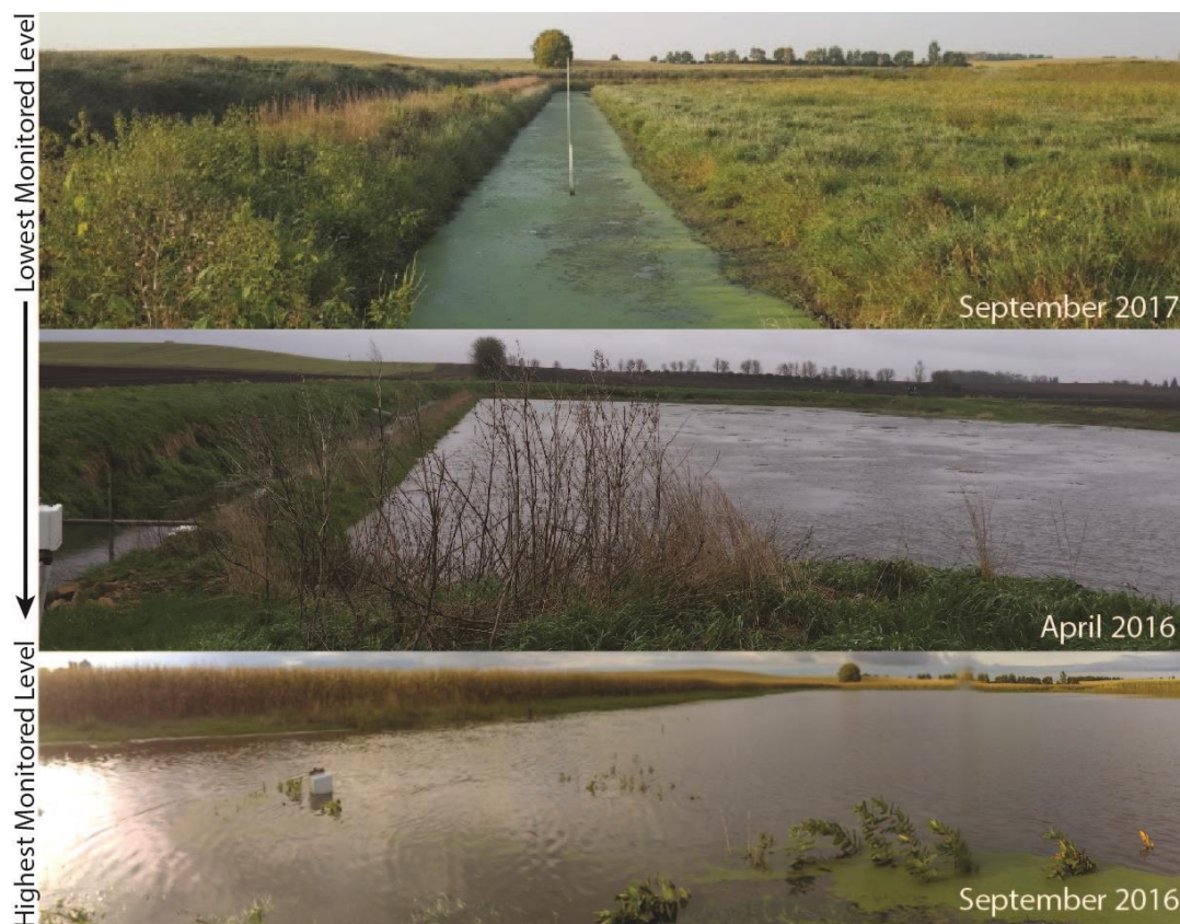
Figure 1.19. County Ditch 57 surge pond and wetland showing lowest monitored, typical, and highest monitored levels on inundation.
