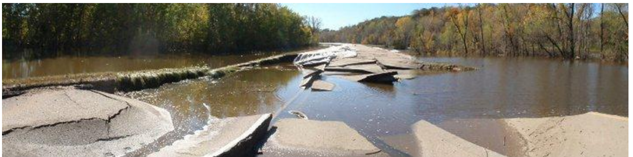
Figure 1.3: US Highway 169 south of St. Peter, Minnesota after Minnesota River flooding in fall 2010
