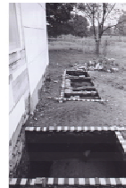
Test pits dug to the rear of the house
