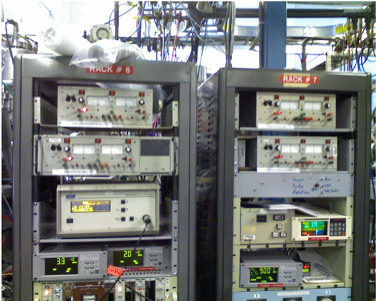
Power supplies, Vacuum gauges, and Gauss meters used in the Merged Beams Experiment
