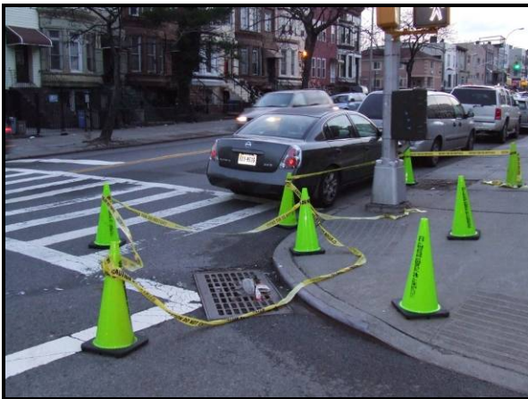
Figure 12. Energized storm drain and traffic light
