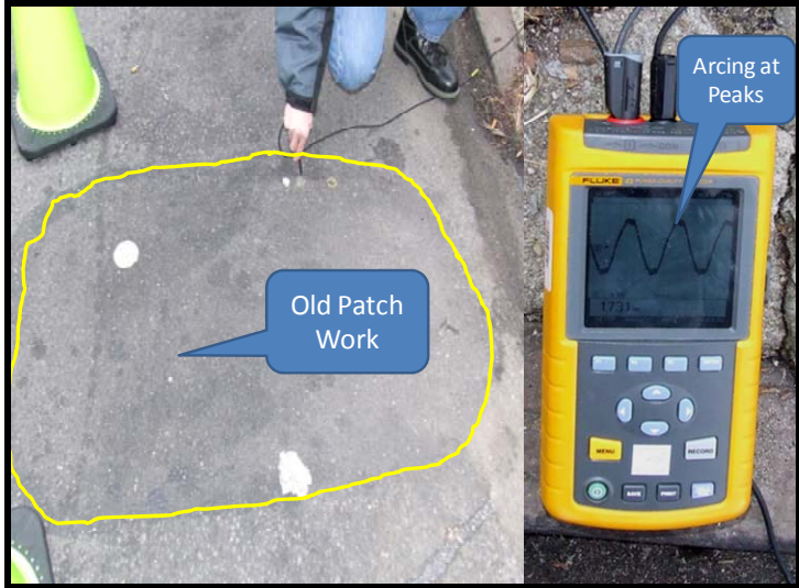
Figure 14. Energized area with arcing verified with Fluke meter
