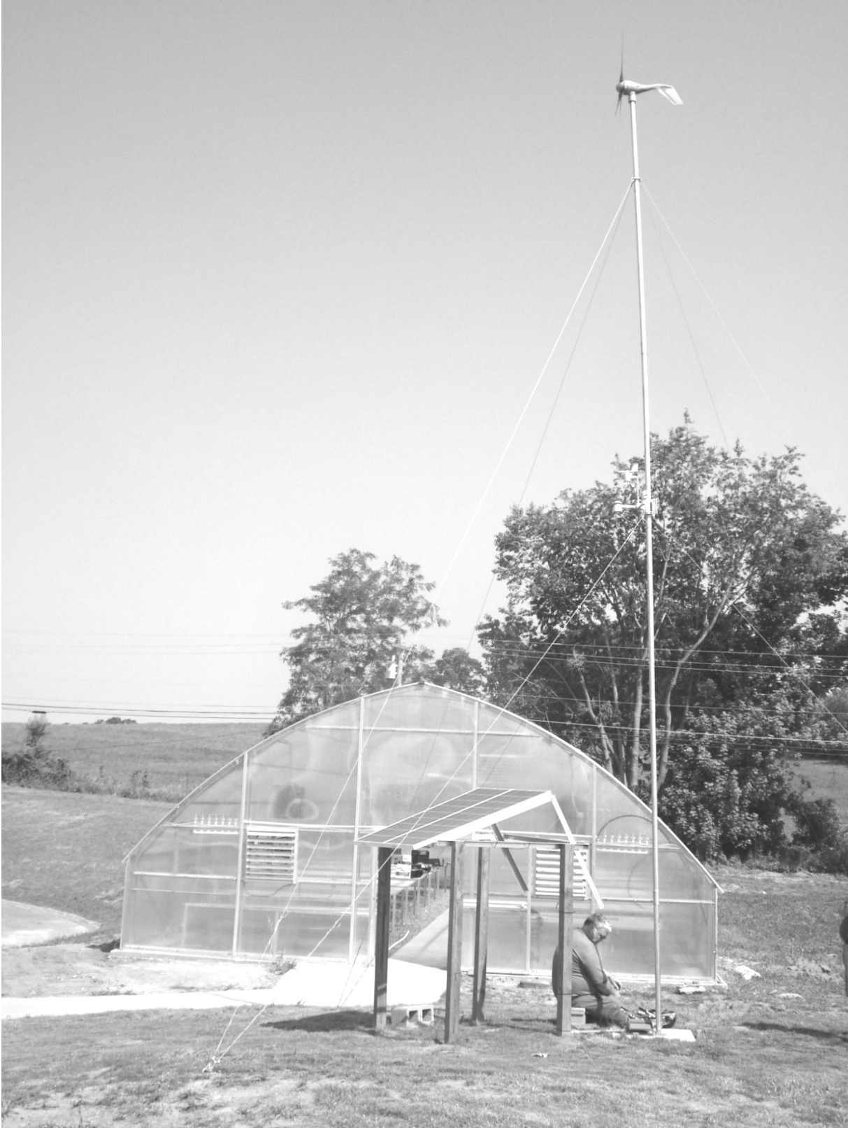
Figure 32. Greenhouse, Turbine, and Solar Panels
