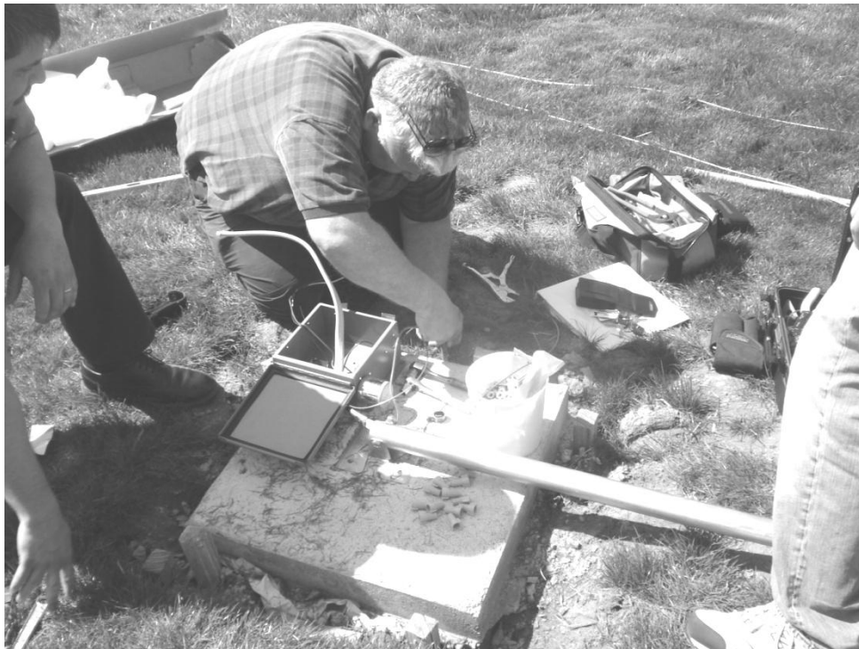
Figure 30. Grounding the Turbine
