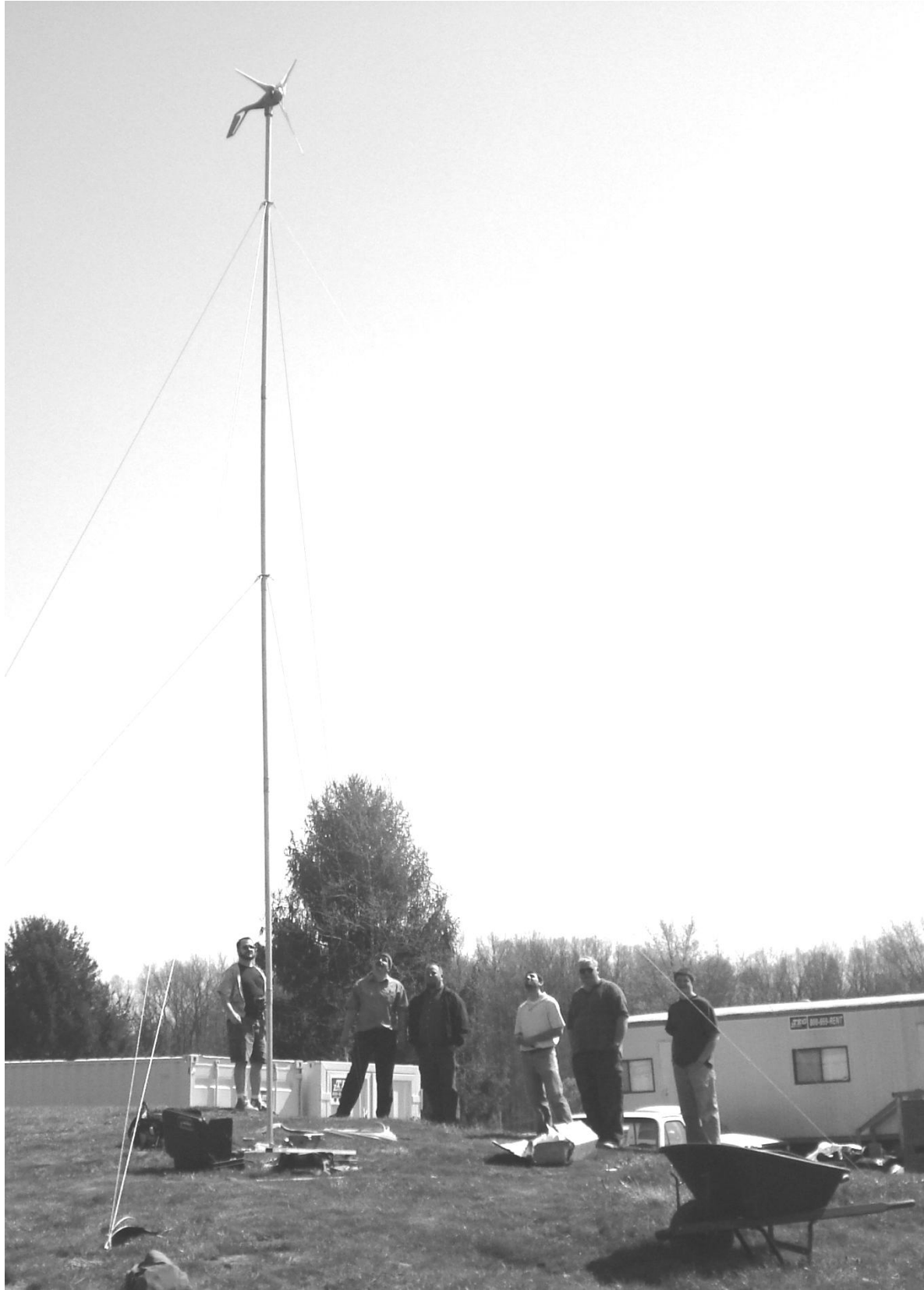
Figure 31. Students and Faculty Erect the Turbine
