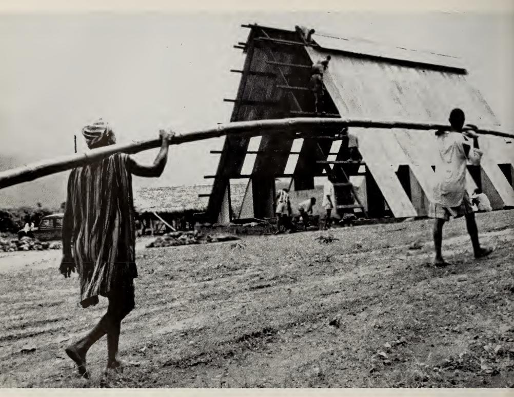
Sierra Leone needed a structure that was inexpensive, comfortable, easy to erect—and able to withstand wind, termites, and heat. The answer: an A-frame designed by VITA members in North Carolina and New Jersey.
