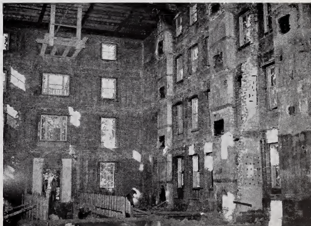
The renovation of Winthrop Hall.
