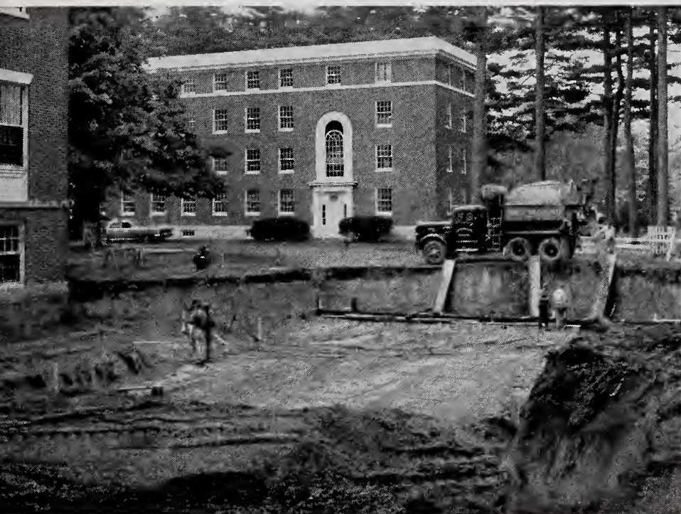
Site for the Moulton Union addition.
