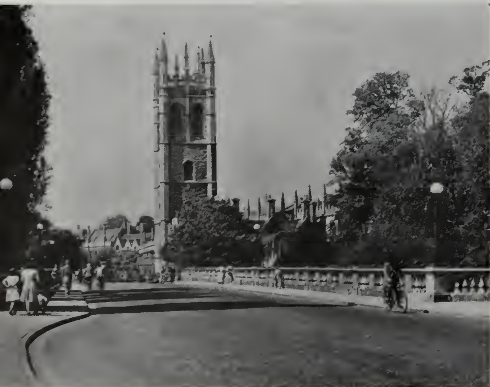
Magdalen Tower and Bridge, Oxford
