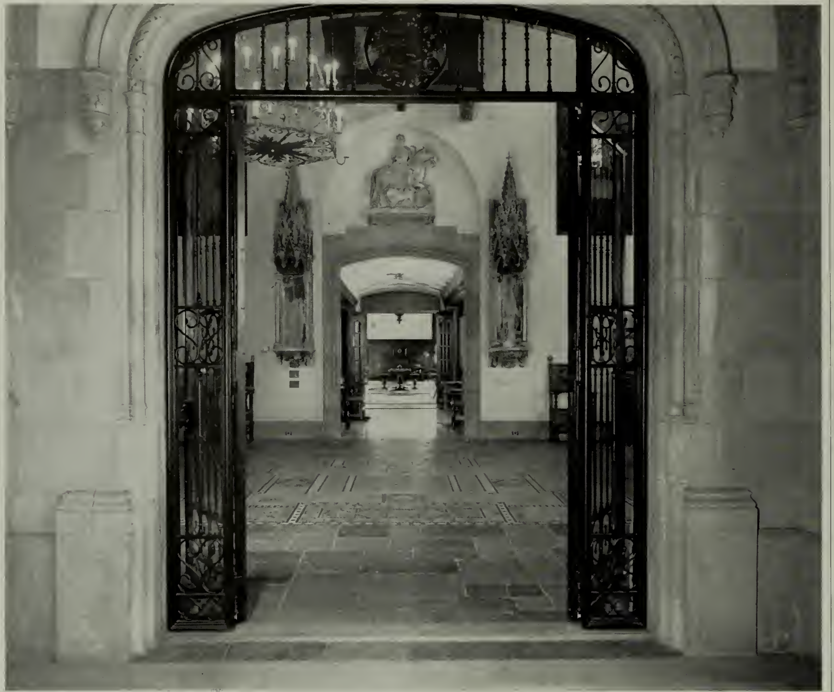
VIEW FROM VESTIBULE THROUGH RECEPTION HALL TO LIBRARY LOUNGE
