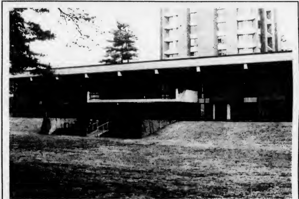
Wentworth Hall is being renovated during the summer of 2000 to triple capacity. The renovations are expected to be complete by that fall. See related story, page 3. (The Fan/Bowdoin Orient)
