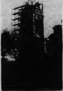
Over one hundred years old, the First Parish Church is currently undergoing a massive face-lift.
