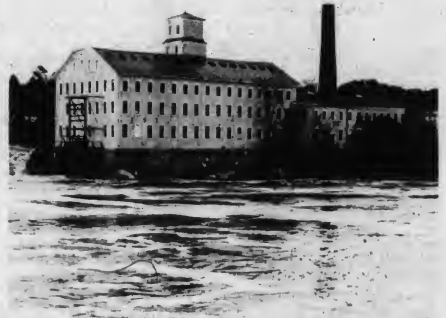
The Pejepscot Paper Mill from the opposite shore of the Androscoggin River. Mills have been a part of the Brunswick scene since the eighteenth century. Orient/Zels
