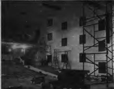
Pickard Theater, the scene of many successful stage and radio productions since its dedication in June, 1955, was a gift of Frederick William Pickard of the Class of 1894. It is shown here in the process of construction.
