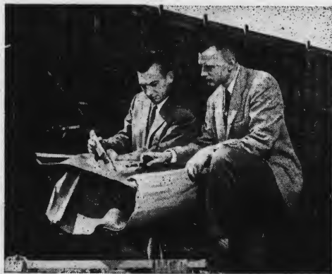
Claire Hruska (left) discusses progress of a new telephone building with the contractor.
