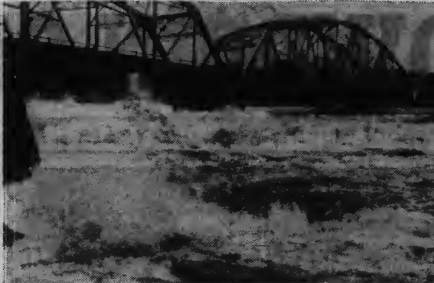
View from just below the Brunswick-Topsam Bridge this shows the swollen Androscoggin River during the flood which hit Maine last week of March. The bridge, closed one day, was itself not actually covered although the Topsam approach to the structure was somewhat washed out.
