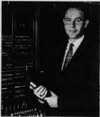
Emmett Smith supervises operation of this training switchboard, which he originally helped to design.
