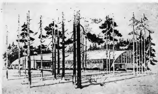
The proposed covered hockey rink to be erected in the Bowdoin Pines.
