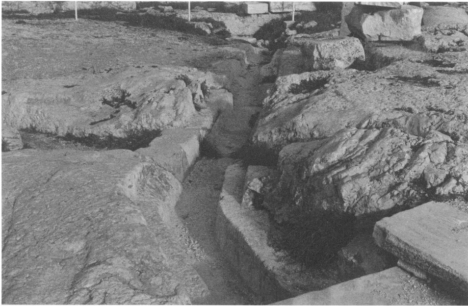
a. Drain cutting leading from the east porch of the Propylaia towards the Archaic cistern. From south
