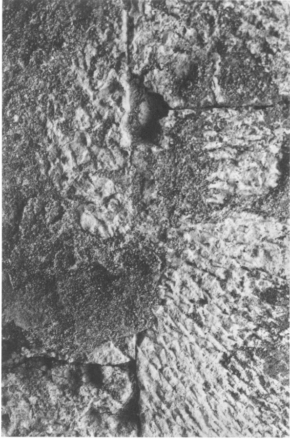
b. Detail of plaster adhering to the cistern wall
