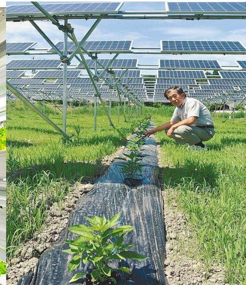
Picture 5. Solar sharing project in Odaka district, Fukushima prefecture
