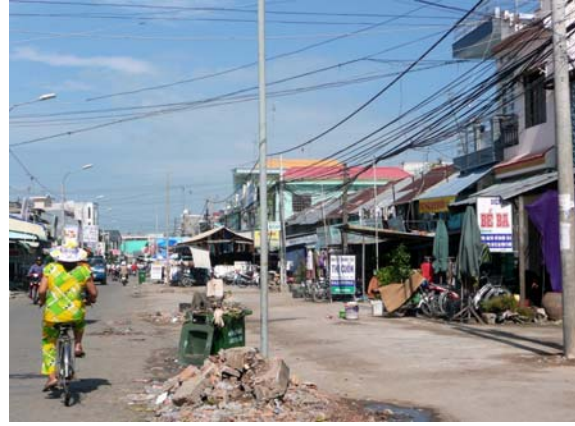
Figure 2: Road along the Thot Not Canal
