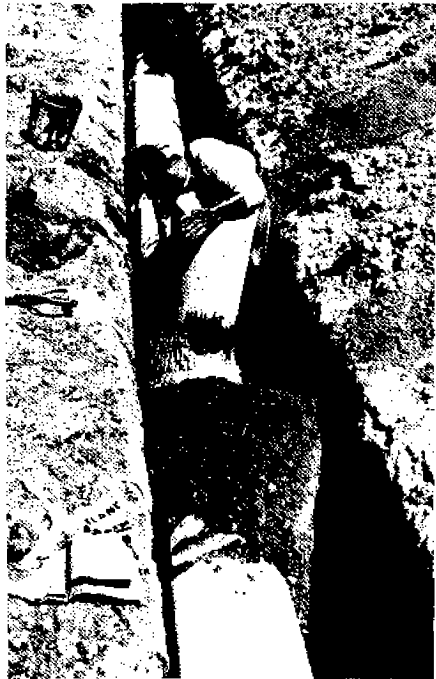
Figure 8.—Prefabricated concrete pipe installation. Riser to accommodate alfalfa valve is being placed.
