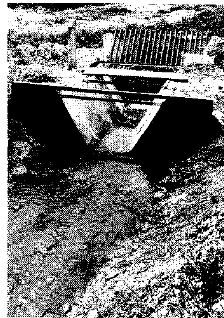
Figure 44.—Trapezoidal measuring flume. In this picture there is also a trash rack downstream on the inlet to an underground pipe system.
