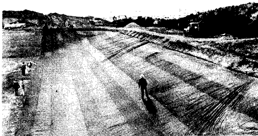
Figure 12.—Vinyl-film lining being installed in a farm reservoir. The section of lining shown is 61 by 300 feet and is fabricated in one piece.
