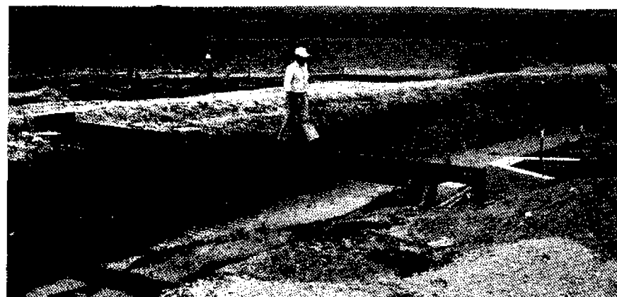
Figure 13.—Two types of flumes used to carry water across ditches and depressions.
