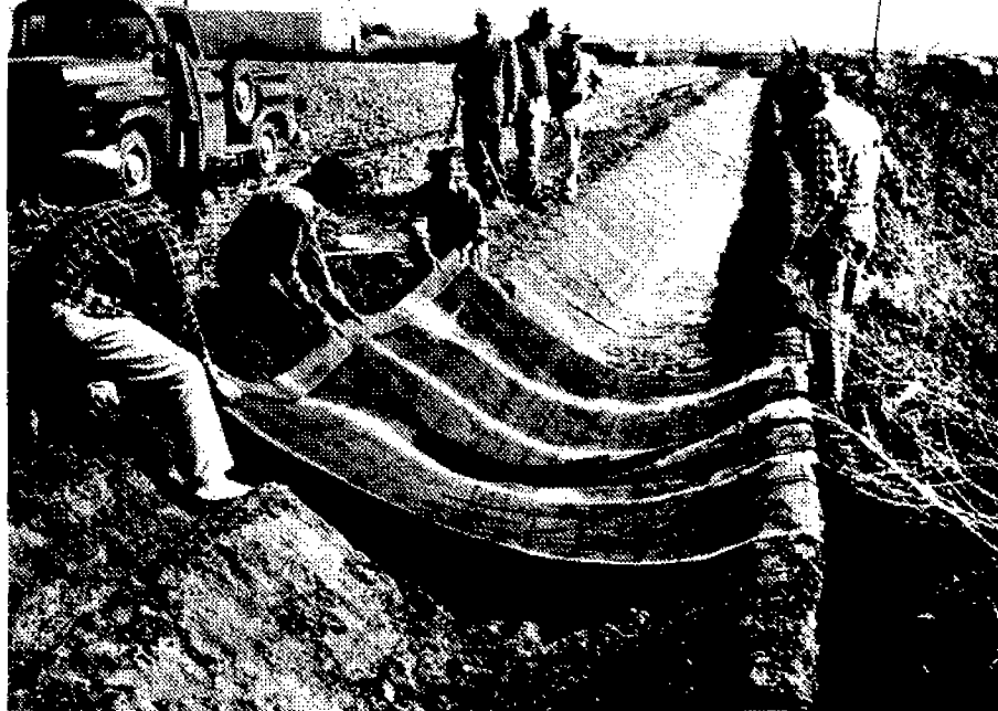
Figure 6.—This asphalt-coated jute liner can be installed by the farmer. The joints are sealed by heating.
