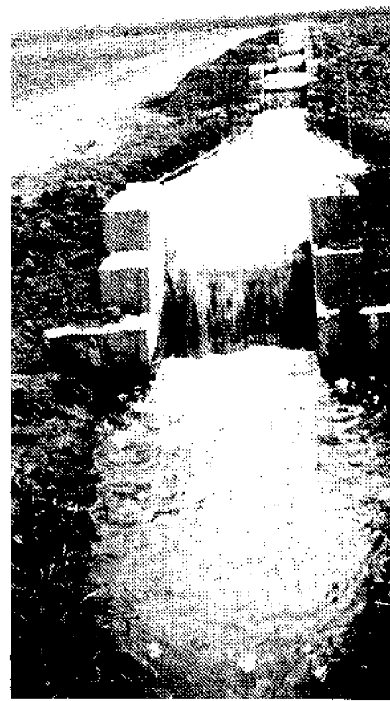
Figure 17.—Concrete-block drop structures being used in an earth ditch. A stilling basin below each drop helps to prevent erosion. BN-16802
