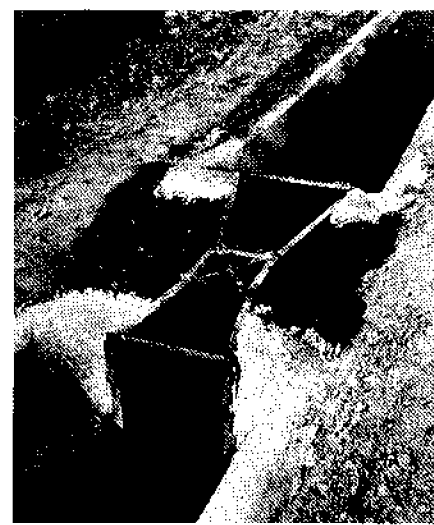
Figure 43.—Parshall measuring flume. These flumes can be constructed of metal or concrete, or of wood specially treated to prevent swelling and rotting.
