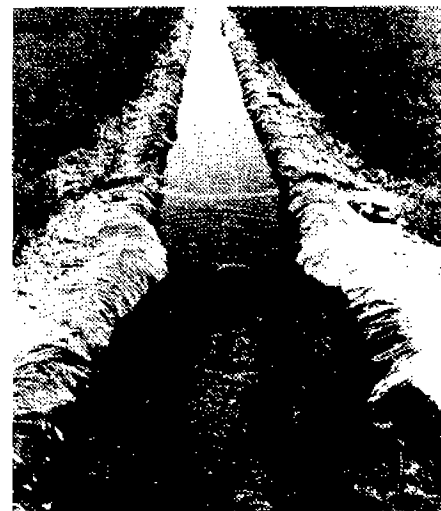
Figure 7.—Ditch lined with polyethylene film. This type of lining is replaced each season.
