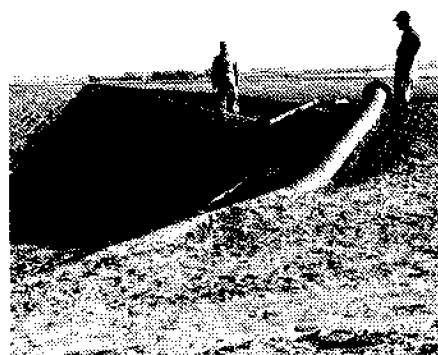
Figure 15.—Built-up, elevated ditches are used for crossing shallow depressions in the field. BN-16812
