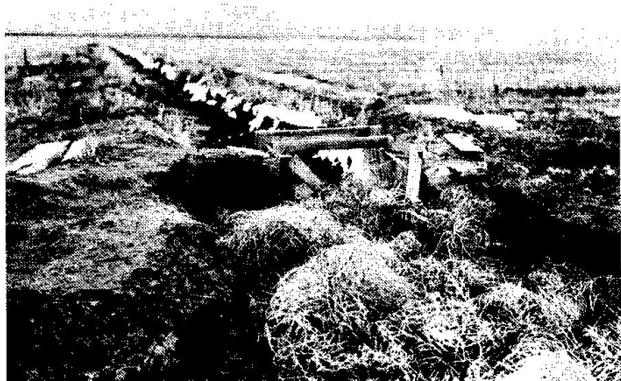
Figure 1.—Irrigation ditch in sandy soil that is badly eroded and filled with weeds.
