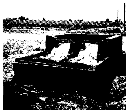
Figure 31.—Debris screen on a gravity inlet to a buried pipeline. This device removes weed seed, is self cleaning, and helps to eliminate the problem of clogging of valves in underground pipe systems.
