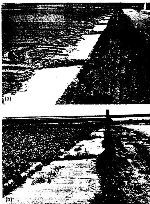
Fig. 2. Buried-pipe erosion and sediment-loss control system. (a) First irrigation after installation. (b) Basins filled with sediment after five irrigations.
