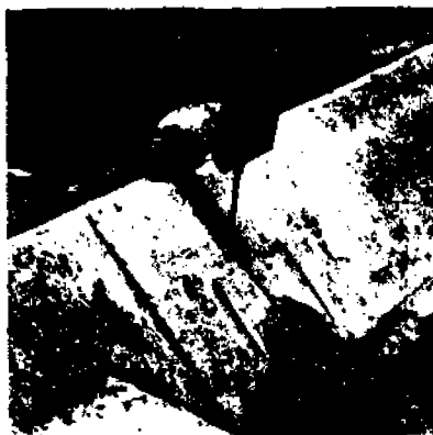
Fig. 6. Drop-closed gate for pipe outlet.
