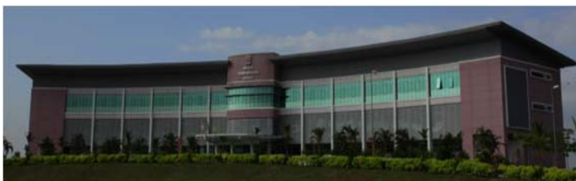
Figure 6 Sepang Municipal Council building
