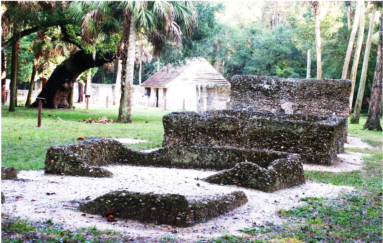
Figure 15: Housing remains constructed of Tabby a concrete made with oyster shells, sand, ash, and water, similar to Coquina (a sedimentary rock), at Kingsley Plantation, Duval County. Photograph courtesy of T. Cavanaugh
