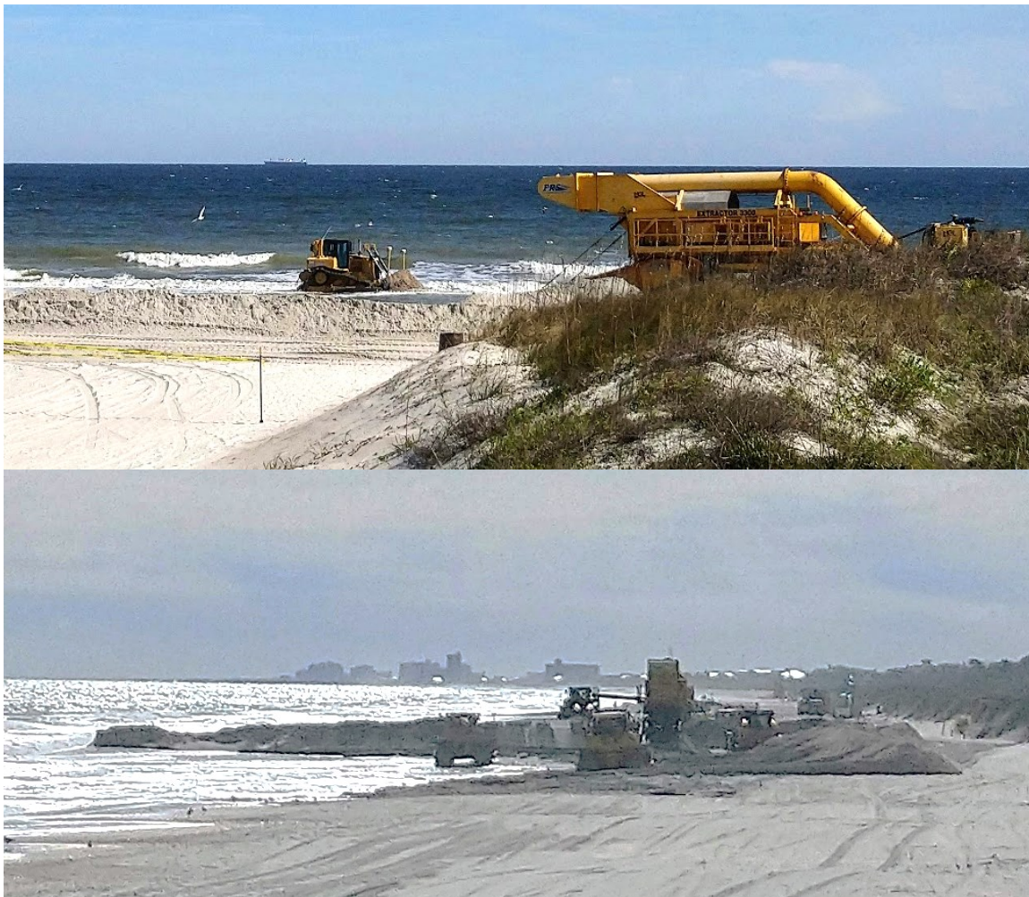
Figure 8: Beach reclamation occurring along the Duval County beaches. Images courtesy of T. Cavanaugh
