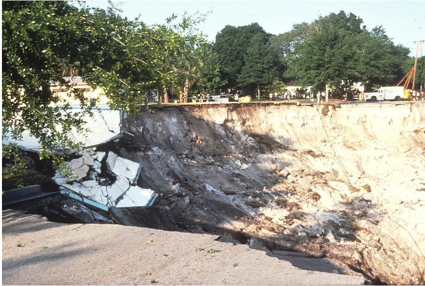
Figure 6: Winter Park Florida cover-collapse sinkhole of 1981. Photograph courtesy of USGS.
