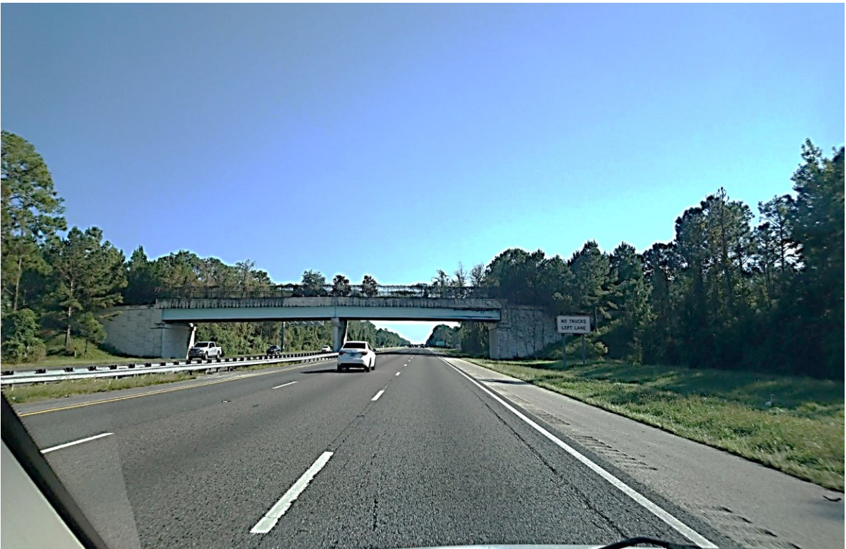
Figure 20: Animal crossing bridge on I-95. Photograph courtesy of T. Cavanaugh.
