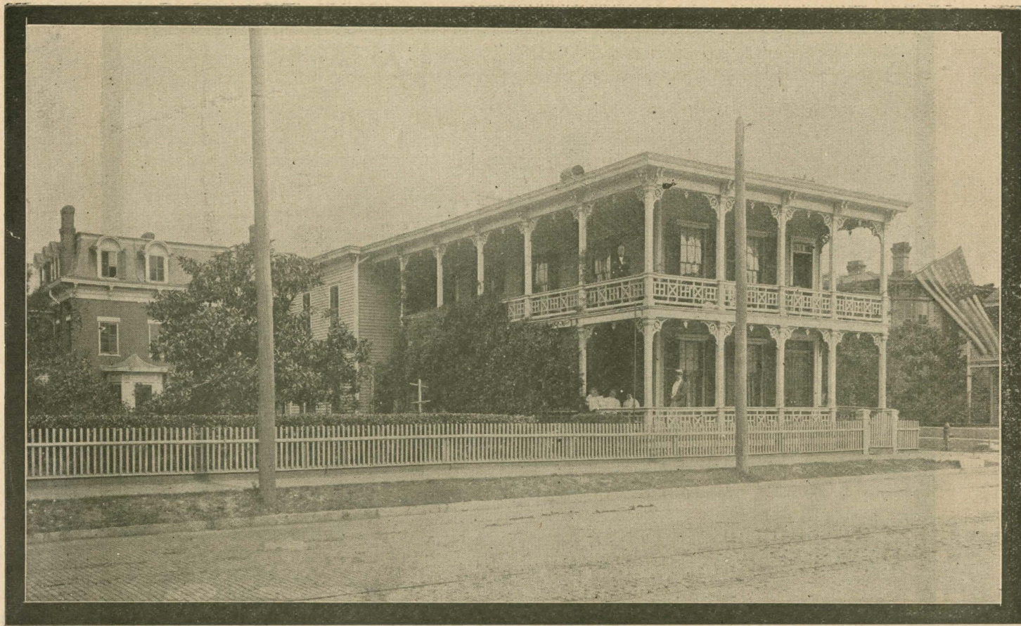
KEENE RESIDENCE—S. W. COR. HOGAN AND ADAMS STREET. A STRAGETIC POINT THAT SAVED A VALUABLE DISTRICT FROM DESTRUCTION.
