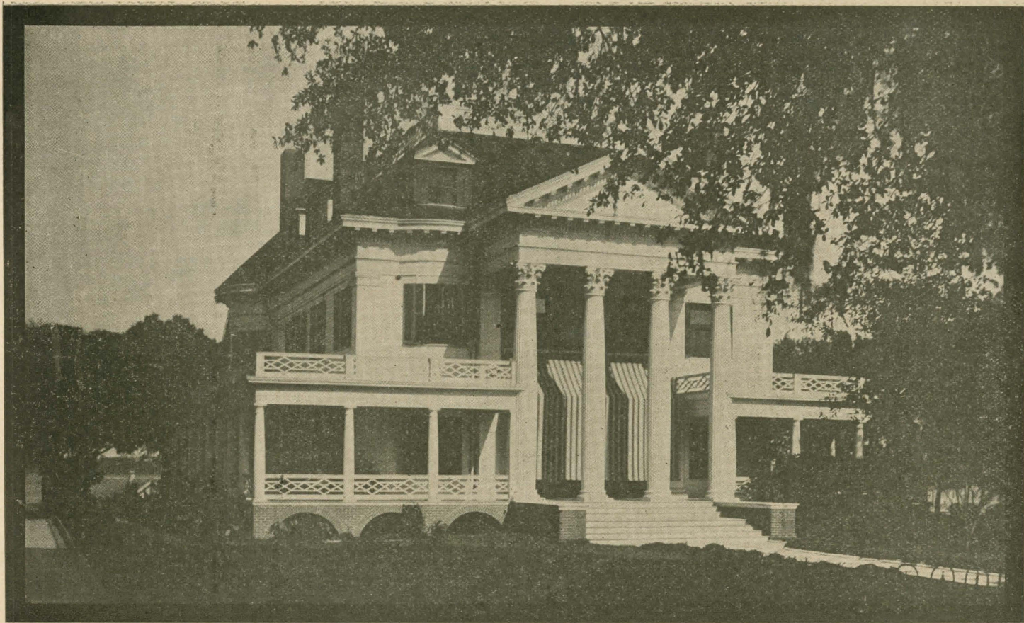
CUMMER RESIDENCE IN RIVERSIDE.
