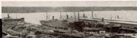
Above... Memorial Park monument. Below... a glimpse of Jacksonville's municipally-owned port terminals.
