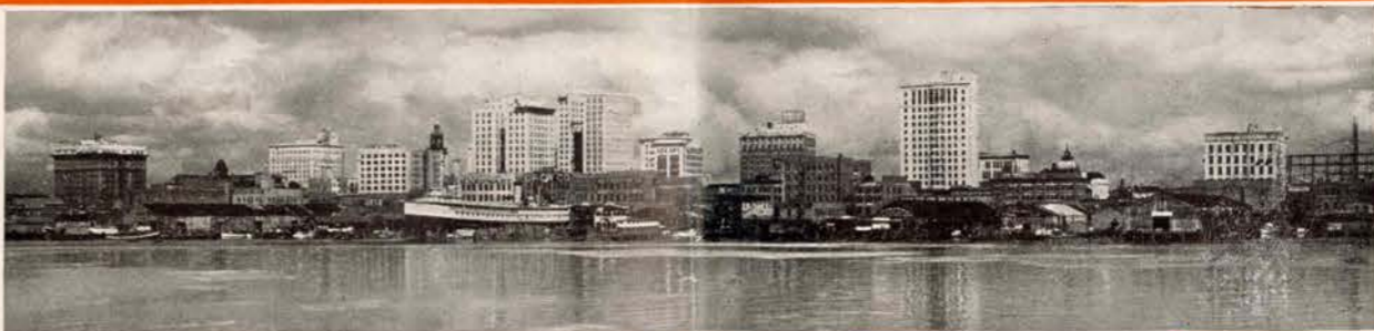
Skyscrapers tower over Jacksonville's golden business district and water-front.
