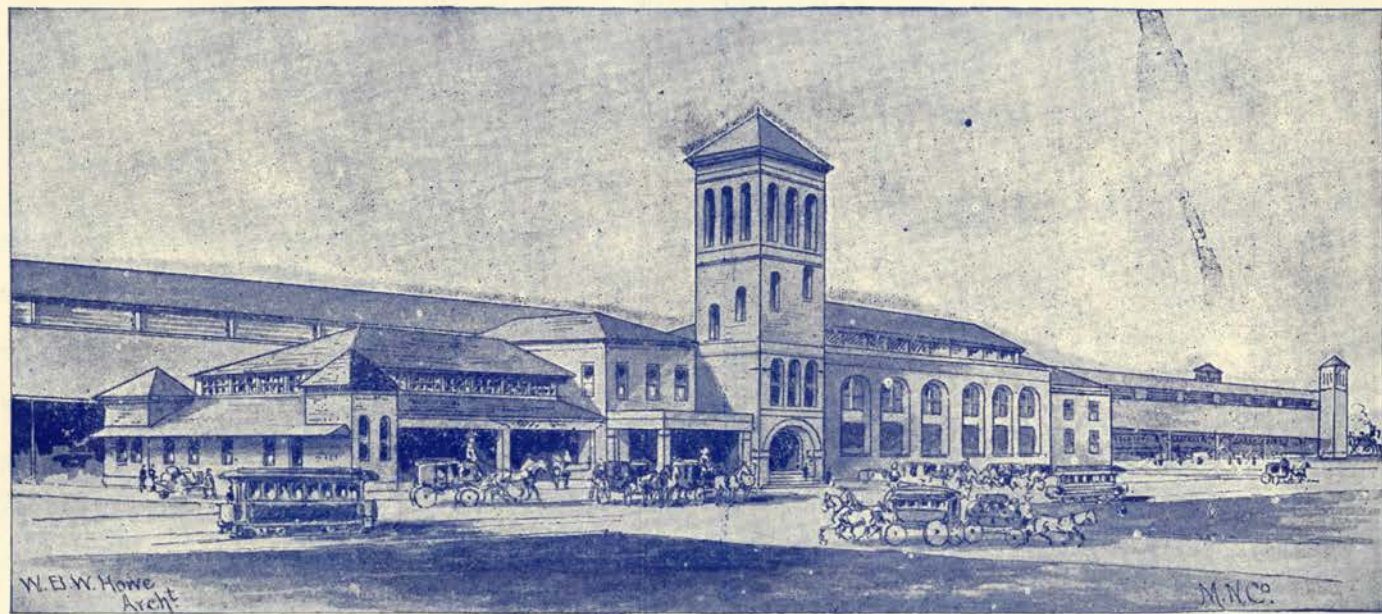
THE NEW UNION TERMINAL STATION, JACKSONVILLE, FLORIDA.
