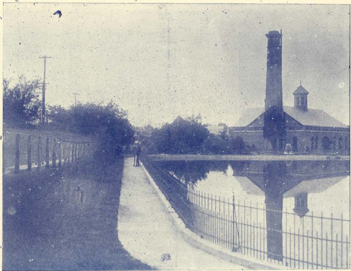
JACKSONVILLE CITY WATER WORKS, FROM WHICH CAMP CUBA USES NEARLY 1,500,000 GALLONS DAILY.
