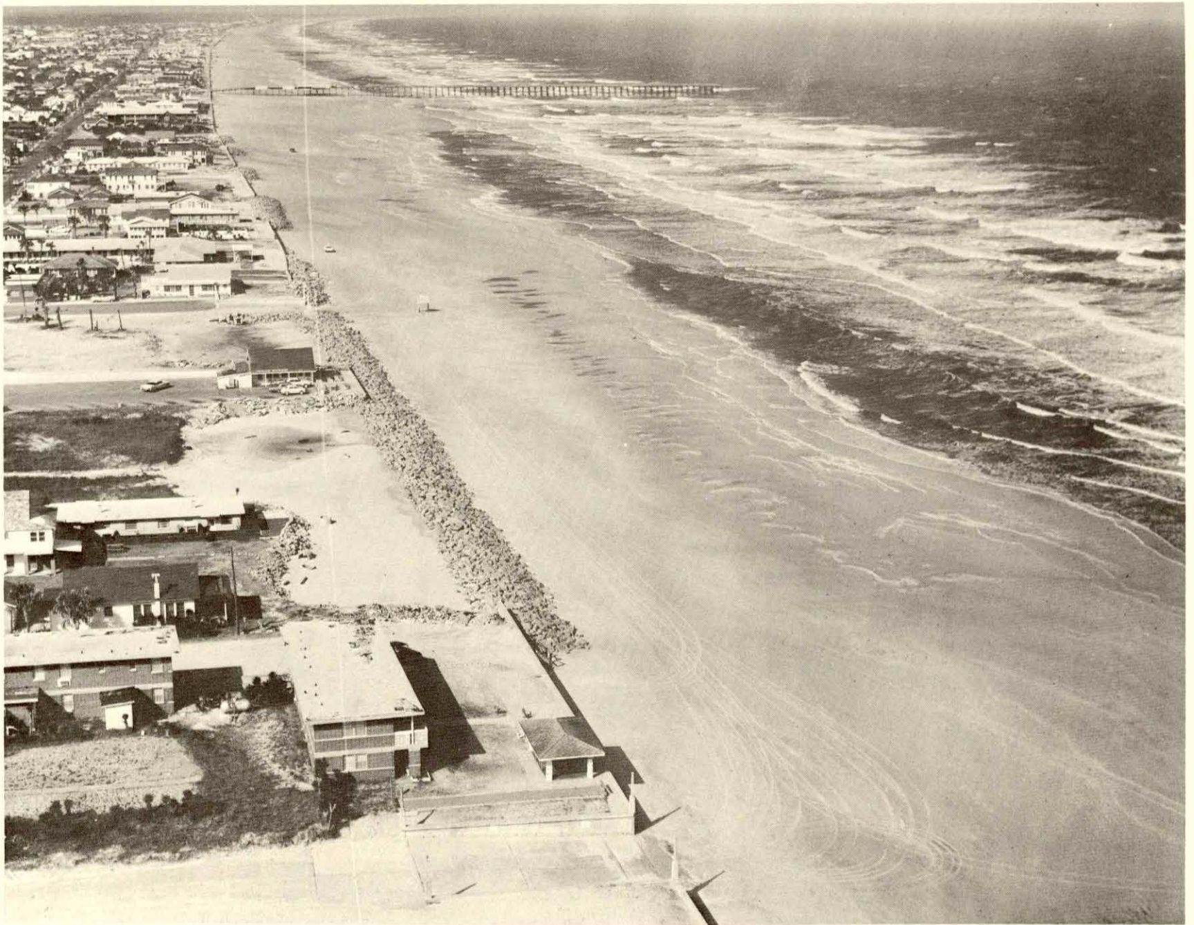
GRANITE REVETMENT AT JACKSONVILLE BEACH (1963)
