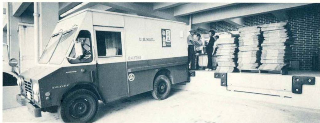
The U. S. Post Office picks up mail four times daily at the new receiving and loading dock located between the 3-story North Building and the West Building Parking Garage. This special ramp was built to accommodate mail trucks which are able to back up to the dock in perfect position for loading and unloading mail.
