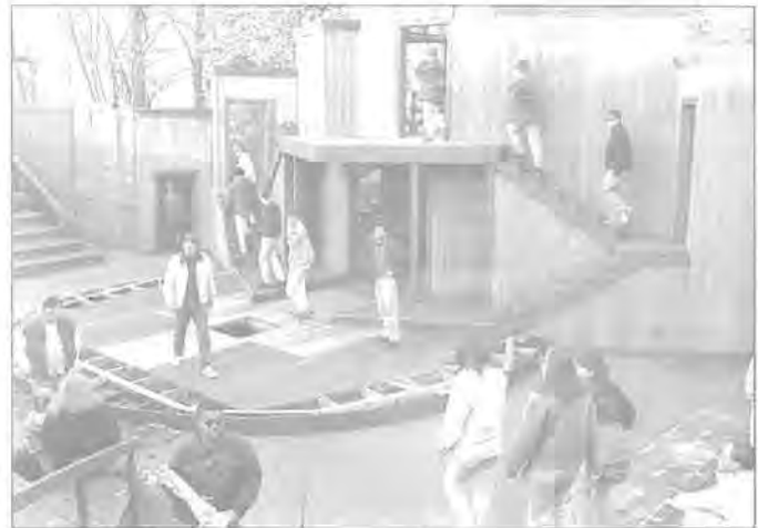
In mid-May, the Company first arrives and begins to explore the stage which will be their home for the next 12 weeks.
