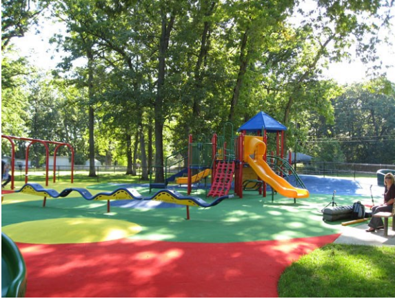
Photo 13: HYB surface system designed with outdoor carpet as top layer over engineered carpet pad base and infilled with silicone sand.
