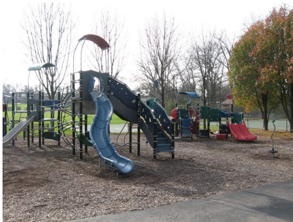
Photo 9: EWF noted with observed undulating surface.
