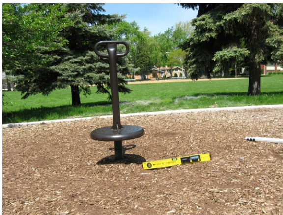
Photo 11: EWF with noted cross slope at ground level play component.
