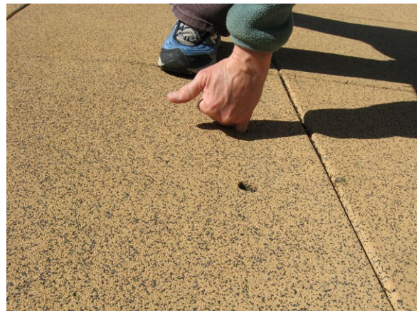
Photo 8: TIL with puncture holes.
