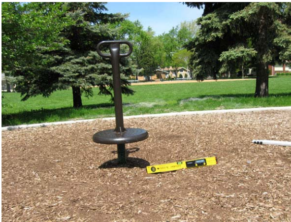
Photo 11: EWF with noted cross slope at ground level play component.
